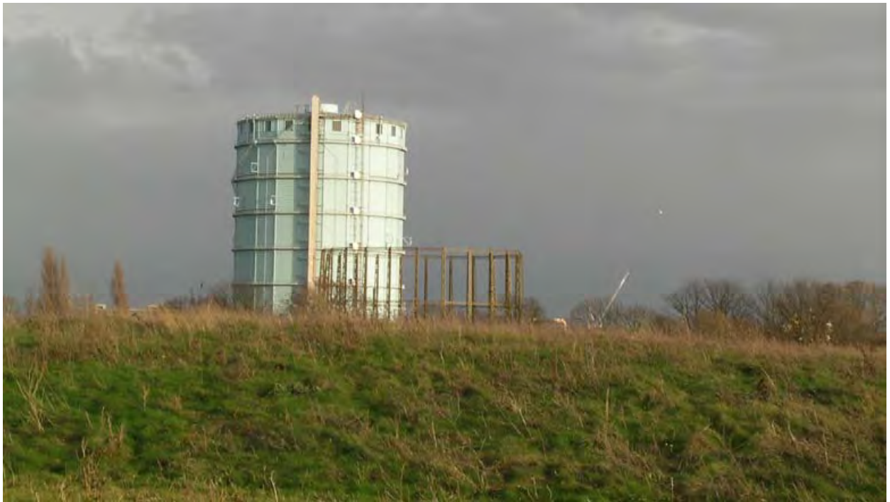
Figure 8. The gasworks site, viewed from the north-west: the box-lattice standards of No. 3 in front of the 'blue tower' fixed gasholder, which is to be retained
