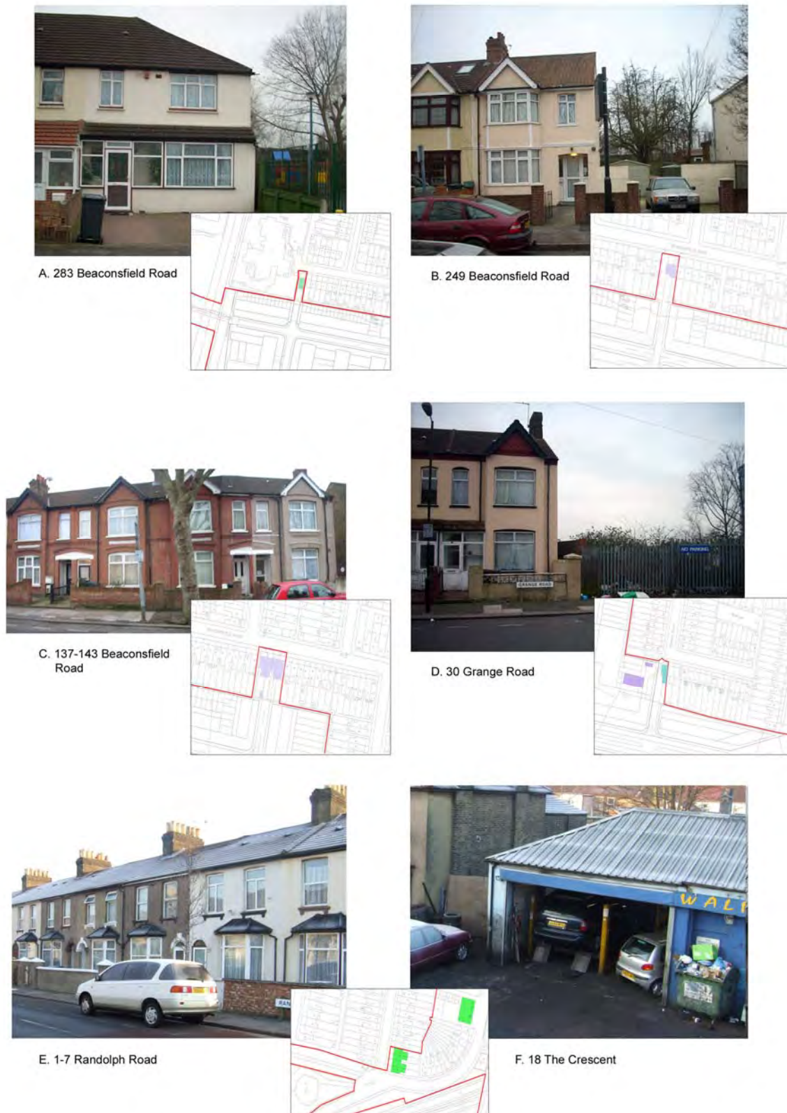
Figure 4. Properties proposed for demolition
