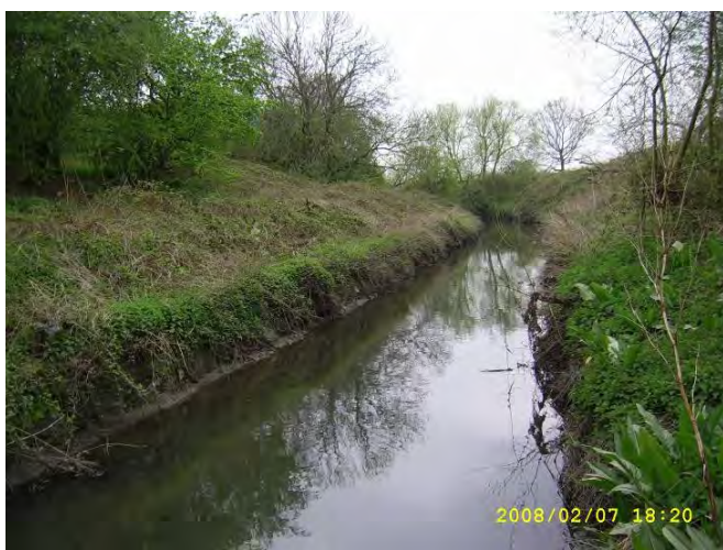
Photograph 3, showing resectioned bank: uniform steep sided bank, straight river channel.
