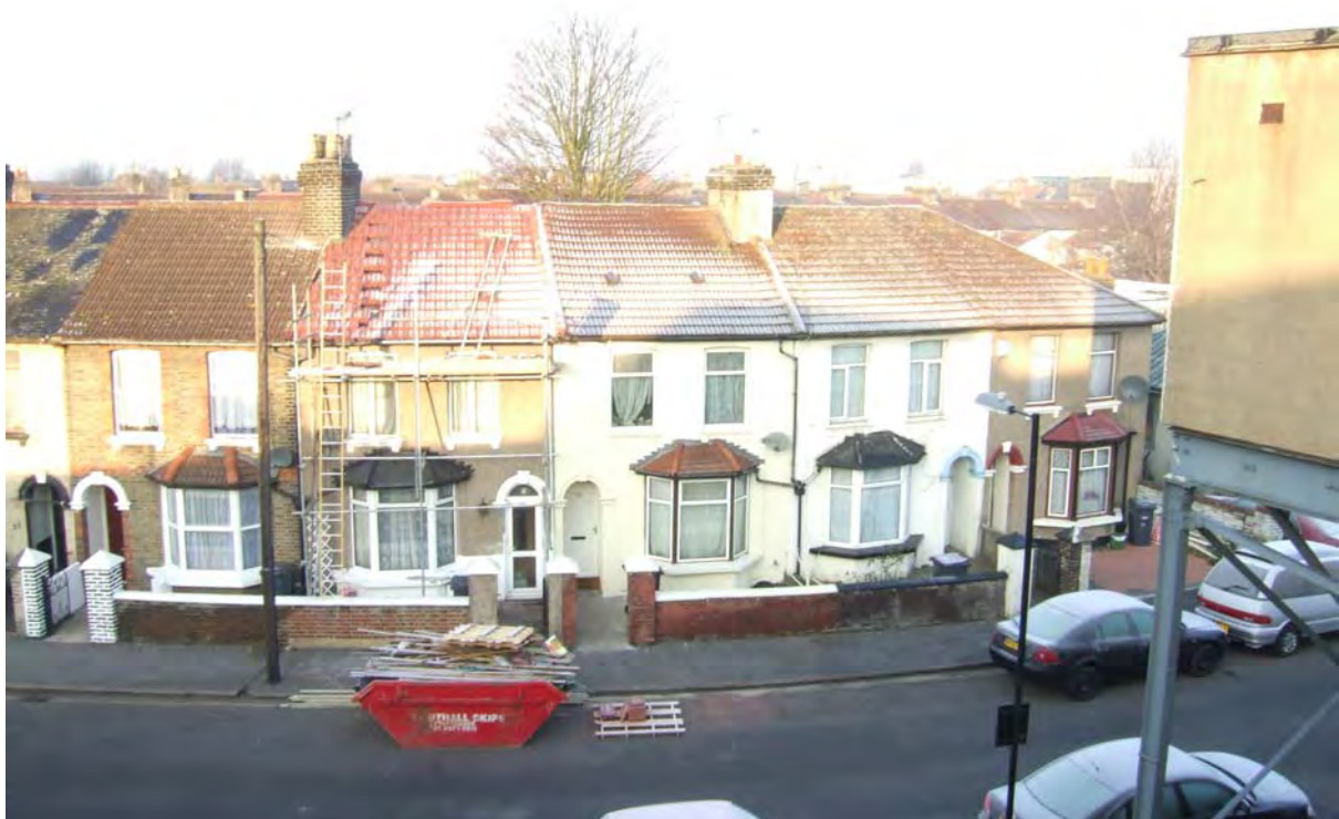
Figure 13. Nos. 20-28 The Crescent, Southall, photographed 20.12.07
