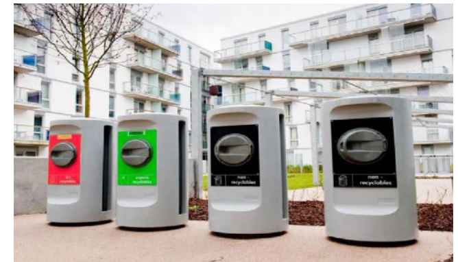
Figure 5.5. Pneumatic waste collection system
