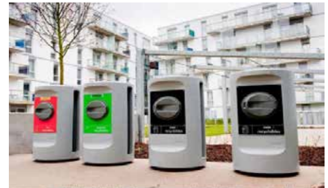
Figure 5.5. Pneumatic waste collection system
