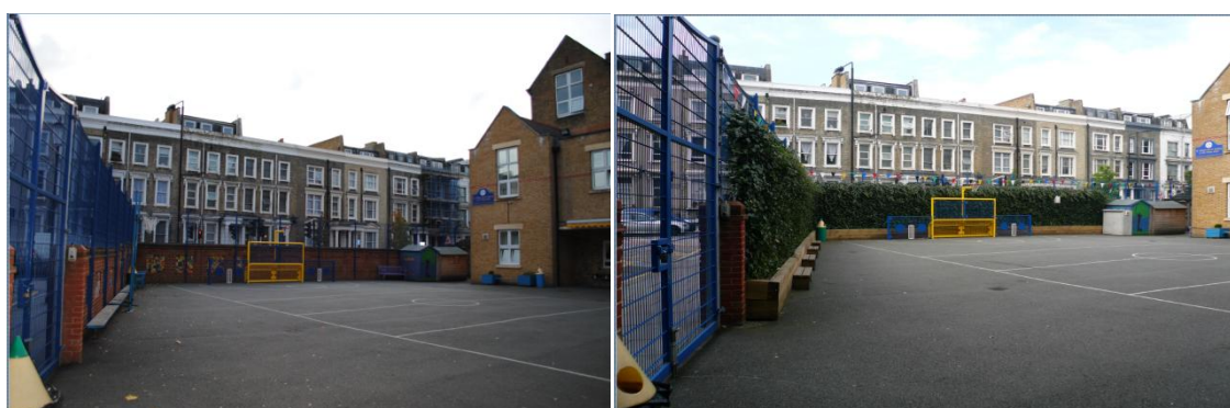
Before Green Infrastructure installation
