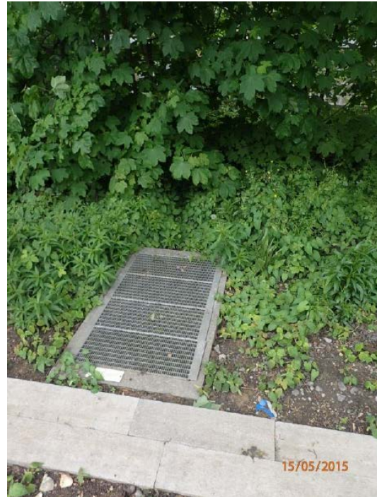
Photo 2: Chainage 580m, looking south. Showing catch pit (M176/CTP2011) located on the shoulder of the East Embankment. This catch pit may require diversion. Taken from Principal Inspection Report of EM4, 15 May 2015.
