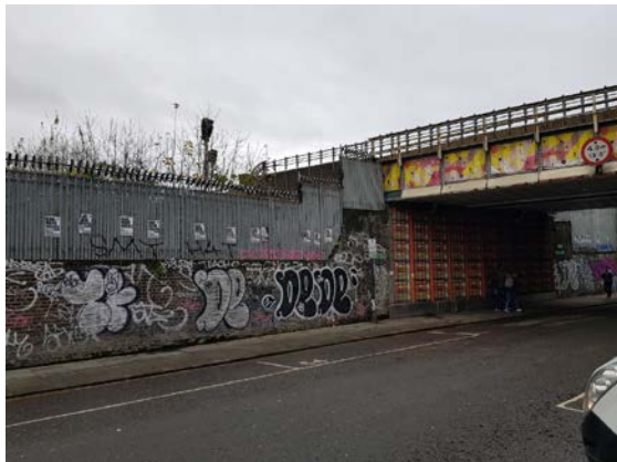
Photo 9: Looking west from Portobello Road. Showing Portobello Road bridge and embankment retaining wall. The embankment retaining wall may be partially demolished once the proposed retaining wall has been installed. The extent of demolition of this wall will depend on the line of the proposed retaining wall taken to avoid conflicting with the Portobello Road Bridge abutment foundations. Taken during site visit on 28 November 2019.
