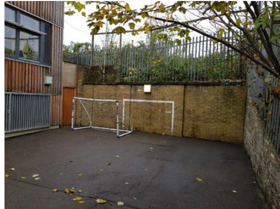
Photo 8: Chainage 640m looking north. Showing the brick retaining wall bordering Notting Hill Preparatory School. Likely to be partially demolished to create development space and to form a connection with the re-entrant length of the proposed retaining wall. Taken during site visit on 28 November 2019.
