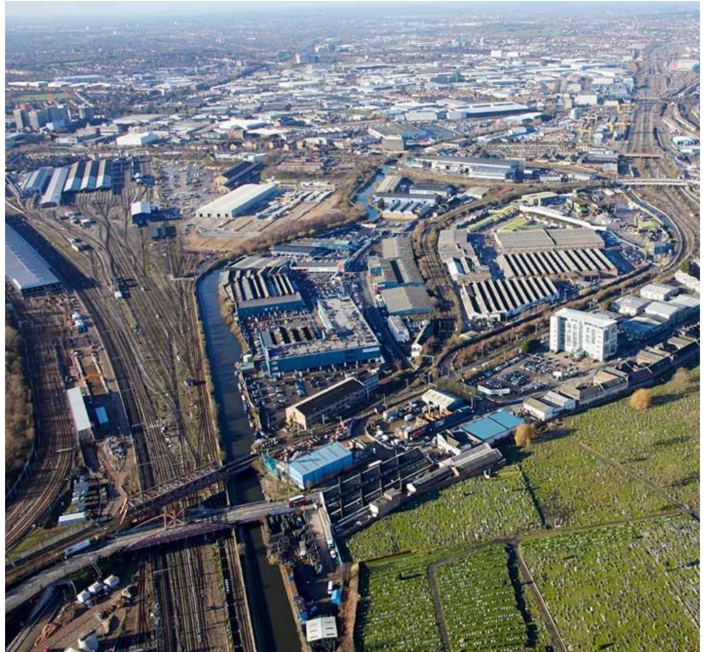
Figure 11.1: Aerial View of Old Oak
