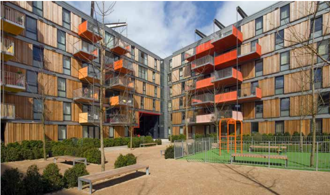
Figure 8.4: Adelaide Wharf, Hackney (credit: Valerie Bennett / AKT II)
