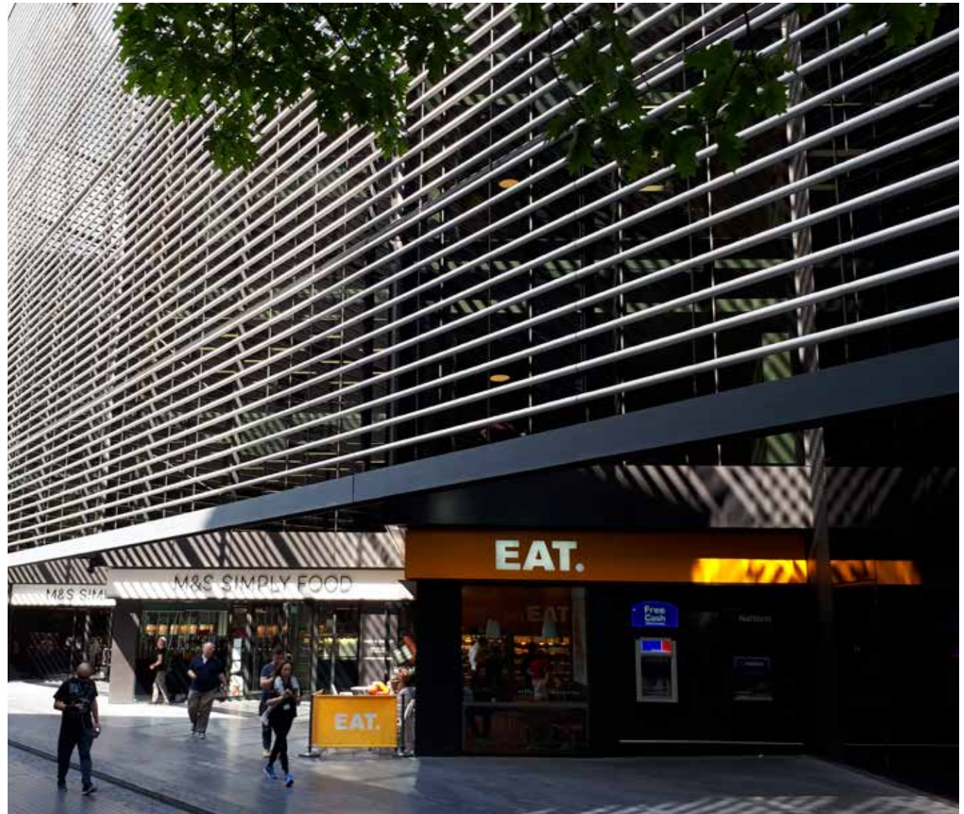
Figure 6.11: High Performance Facade, More London
