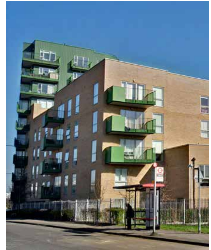
Figure 4.20: Recent residential development within Park Royal Centre
