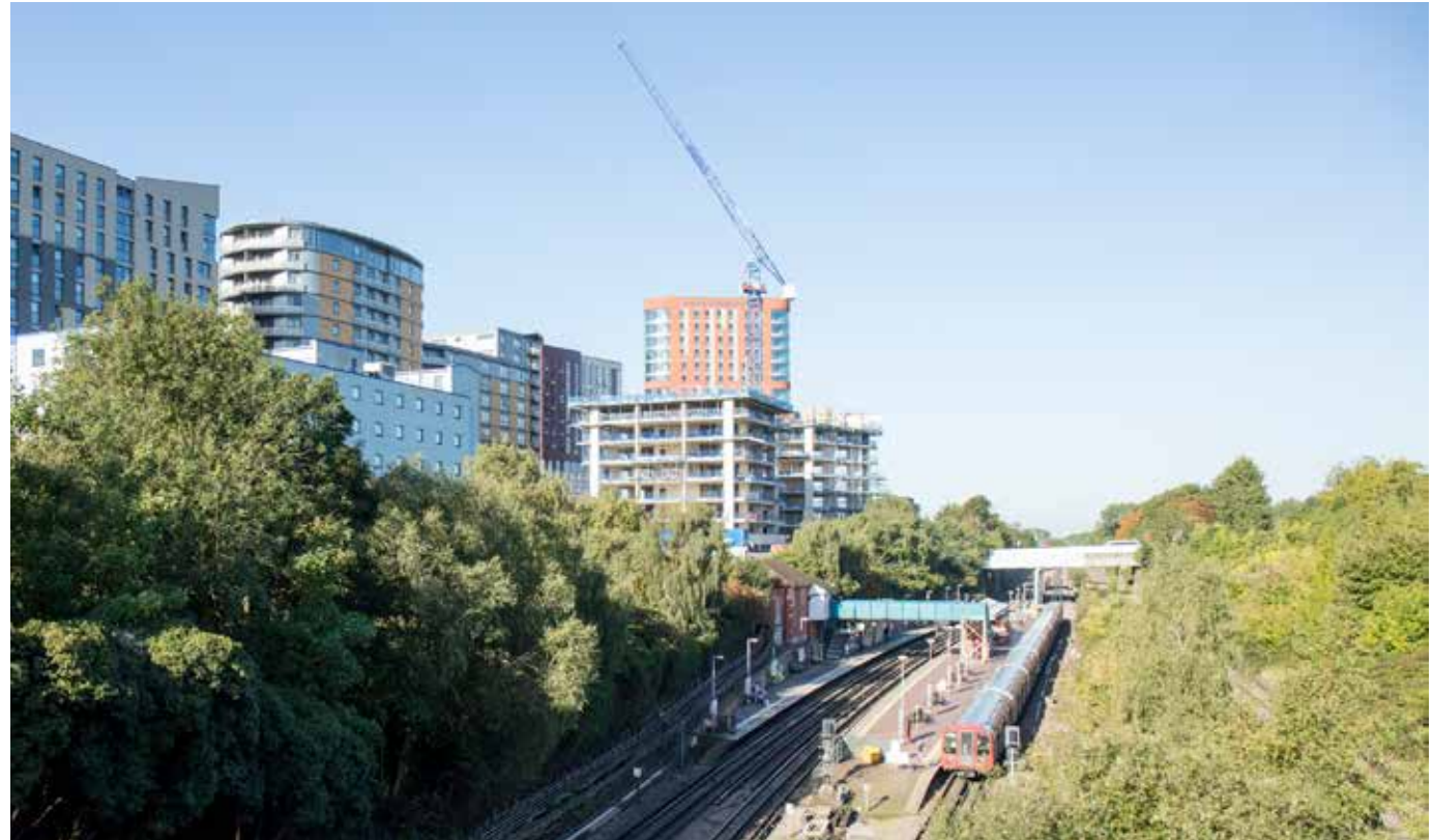
Figure 4.24: North Acton Station
