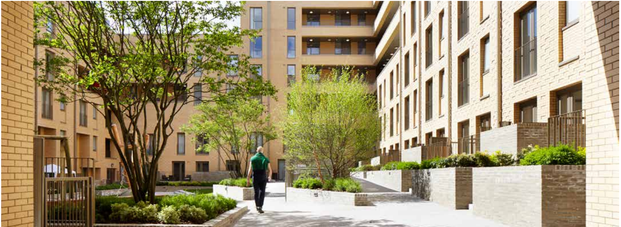
Figure 8.1: St Johns, Clapham (credit: Jack Hobhouse)
