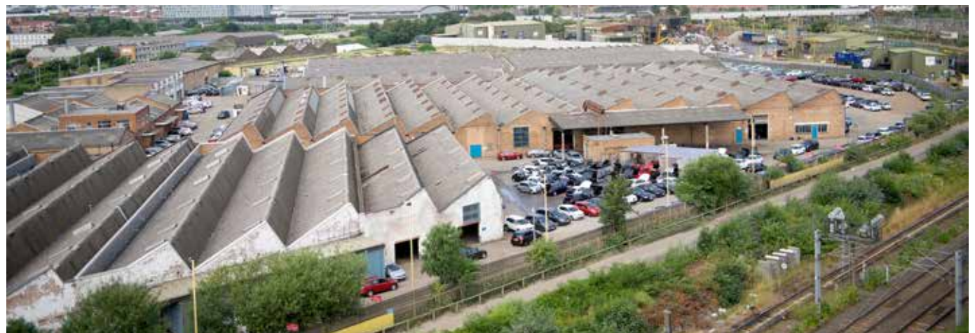
Figure 4.8: Existing industrial character of Old Oak North
