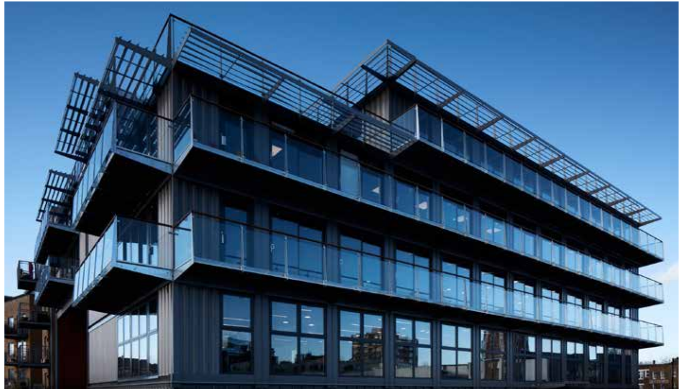
Figure 6.10: Recycled Shipping Containers, Roundhouse, Camden (credit: Furness Partnership / Tom Carter)
