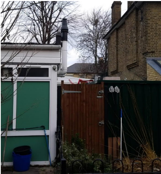
Boiler flues of older section of building and air heating system in new section
