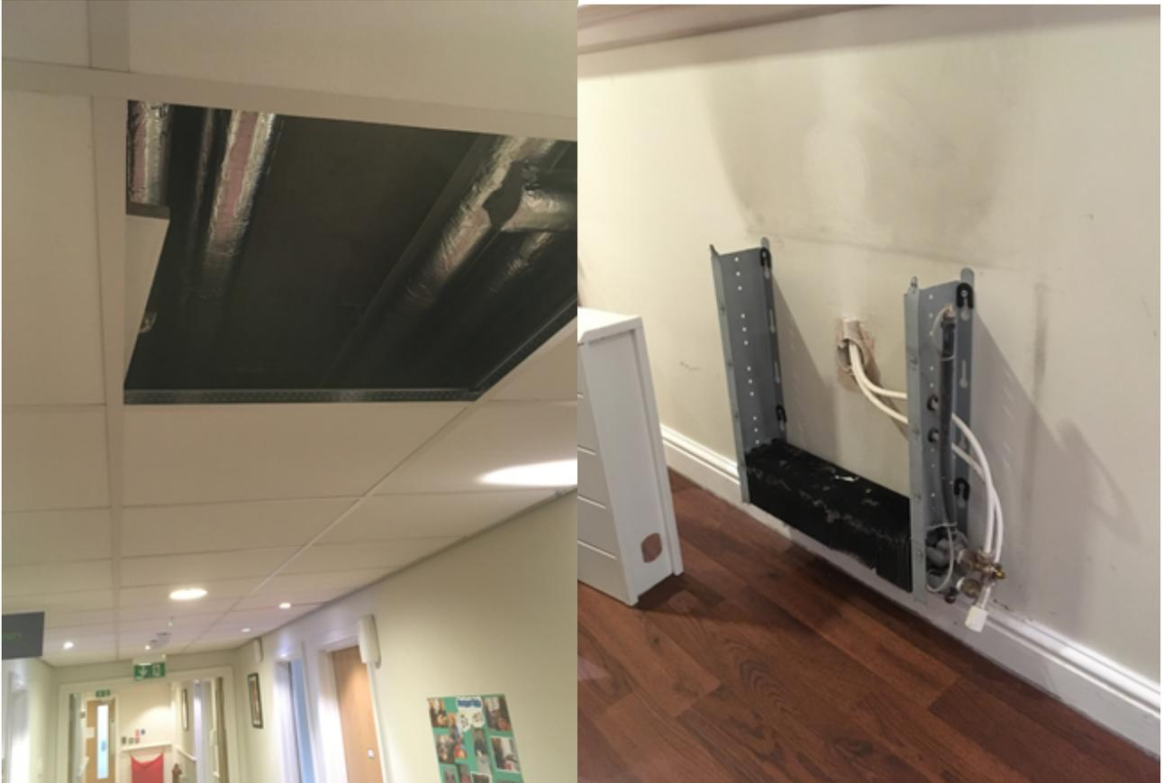
**Figure 6. Corridor ceiling showing insulated piping (left) and corridor radiator (right). All radiators have heating element at the base, with a large casing above to reduce the risk of residents burning themselves.**
