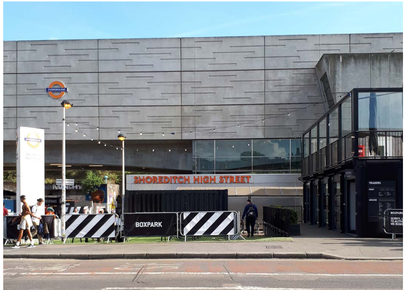
Figure 4.26: Shoreditch High Street Overground Station
