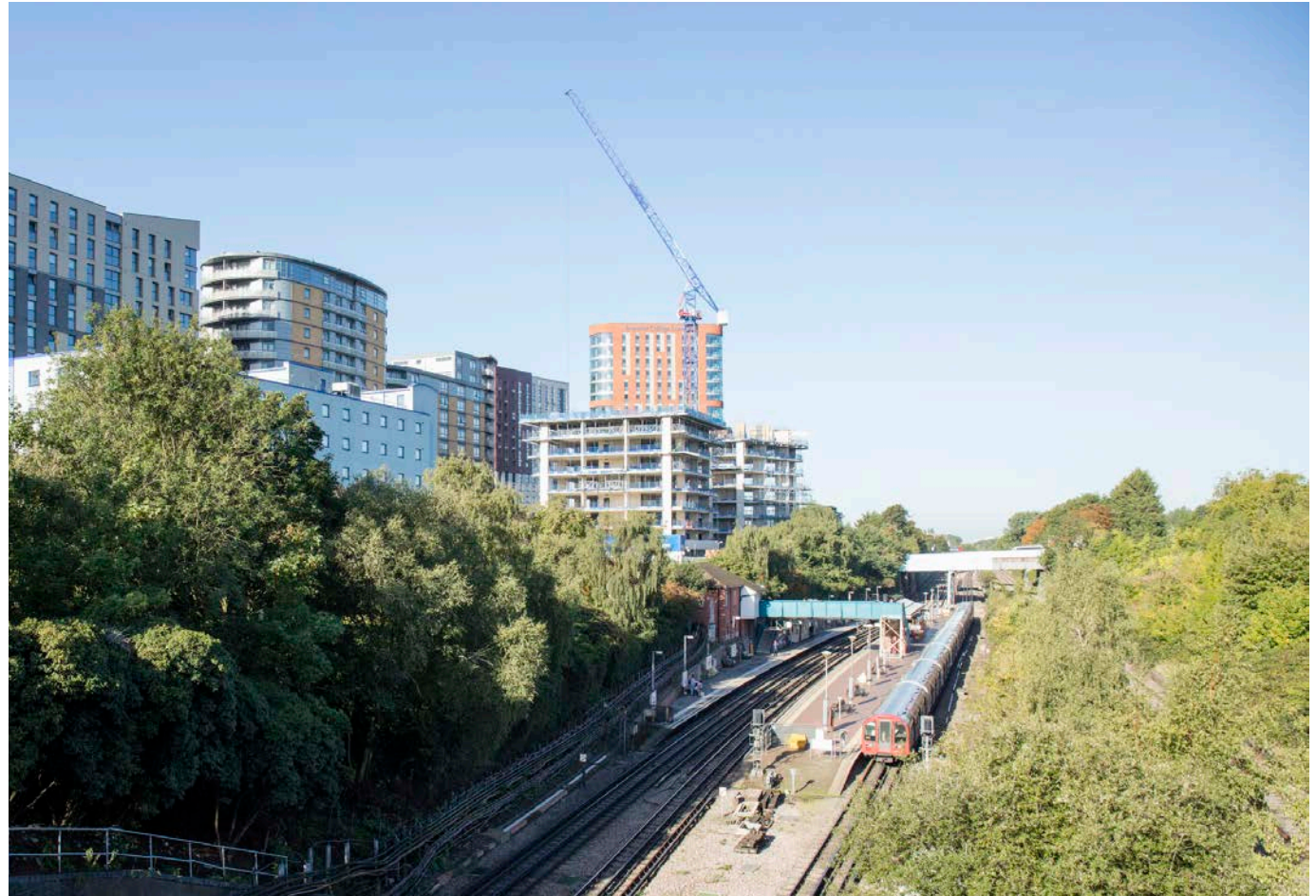
Figure 4.24: North Acton Station
