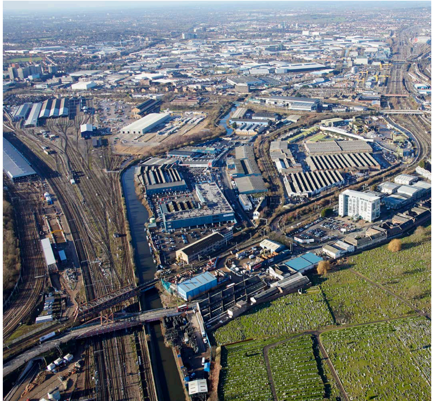
Figure 11.1: Aerial View of Old Oak
