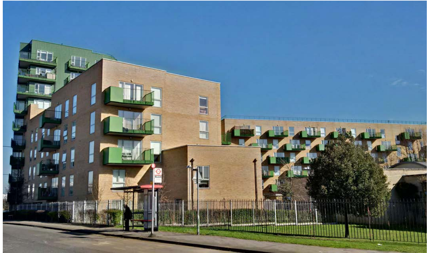
Figure 4.20: Recent residential development within Park Royal Centre
