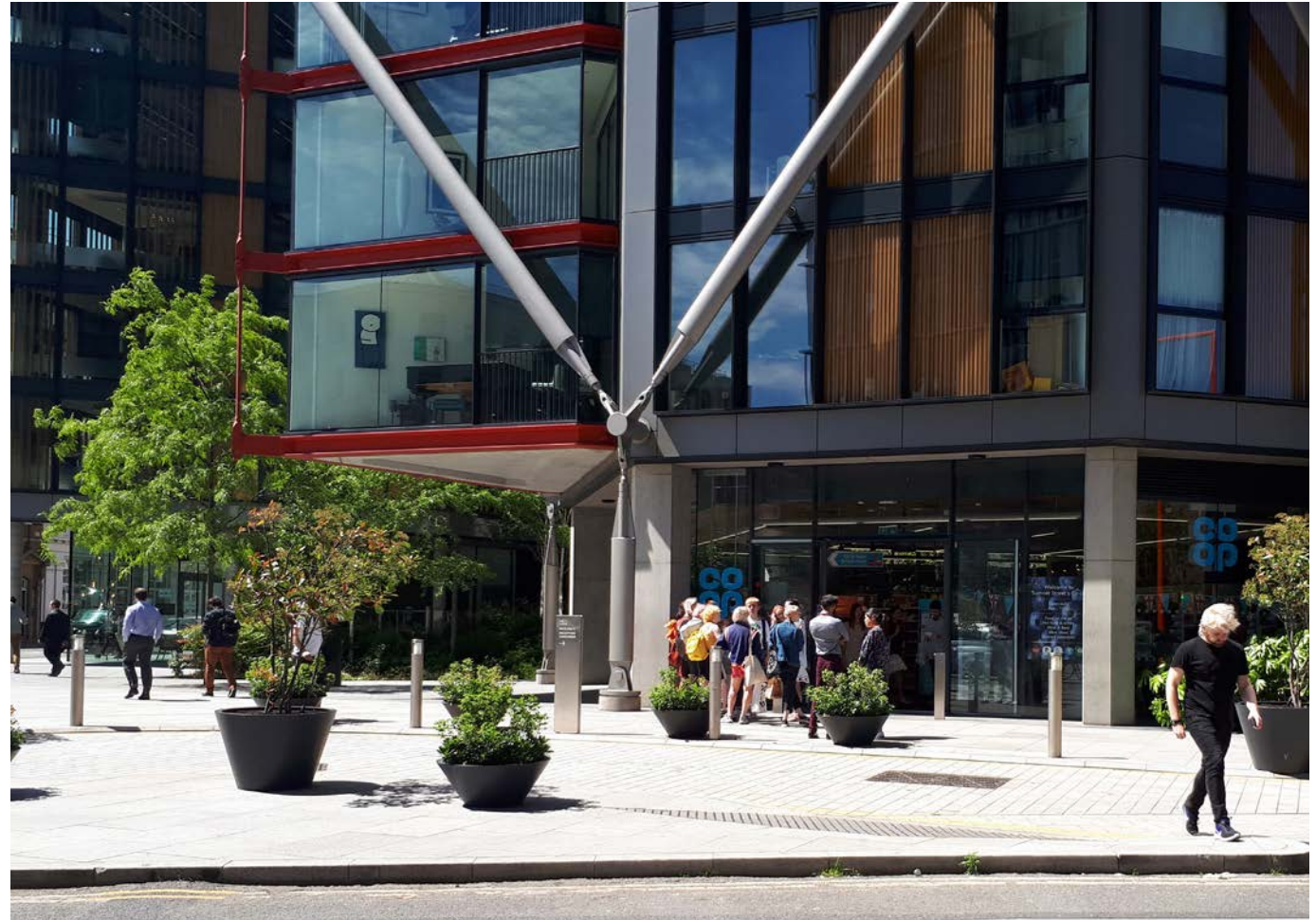
Figure 4.39: Neo Bankside, Southwark Street, London
