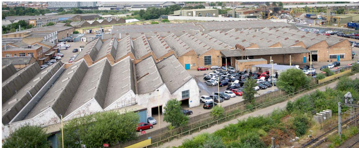
Figure 4.8: Existing industrial character of Old Oak North
