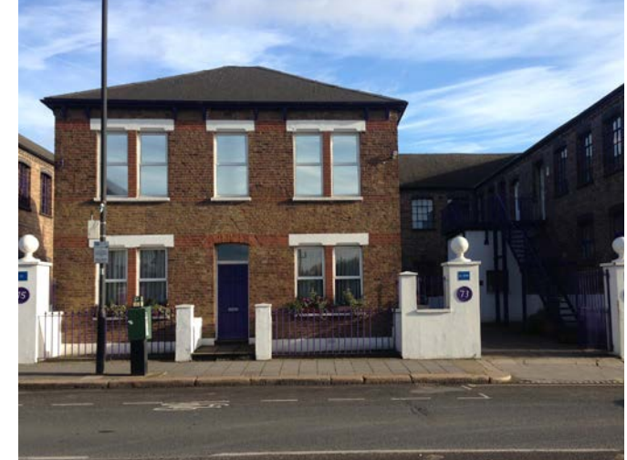
Figure 4.35: Cumberland Park Factory, Scrubs Lane
