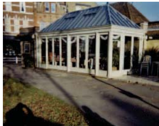
Former public toilet – now café, Richmond
