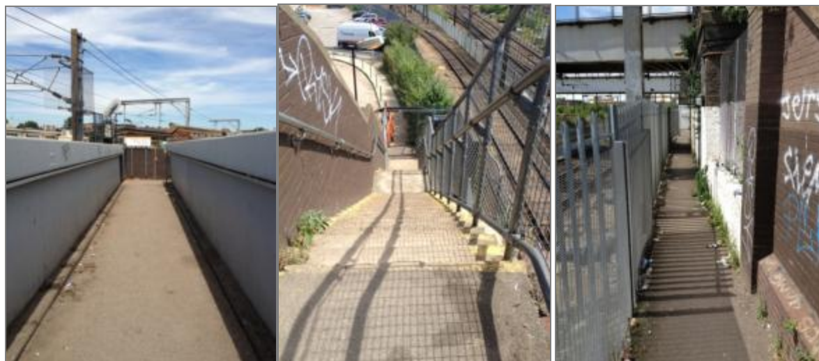
Figure 4-13: Current pedestrian access to Willesden Junction station, from the south
