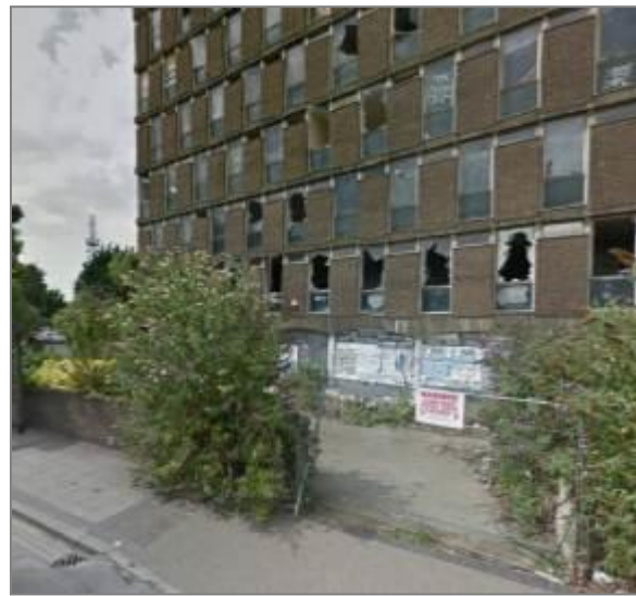
Figure 4-24: Derelict building located on Old Oak Lane.
