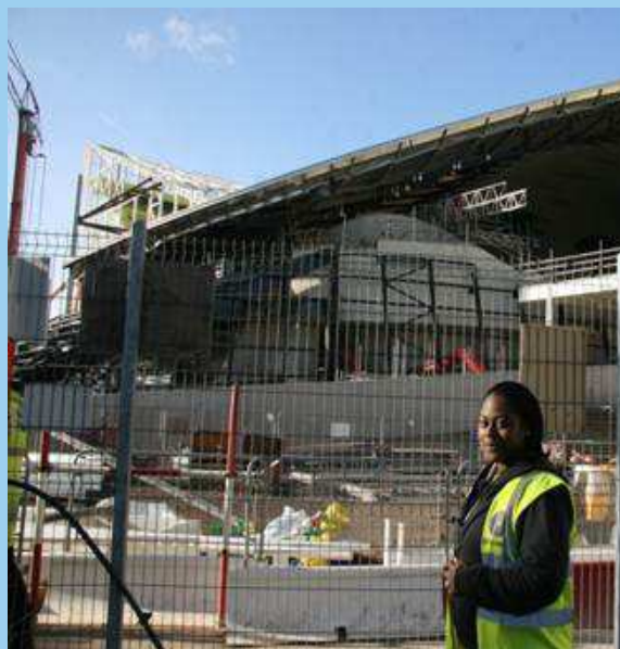
Jadene working on the Aquatics Centre
