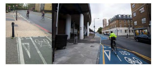
Problem: lack of priority across side road, and inappropriately wide side-turning geometry. L: South Lambeth Rd; R: Cable St.
