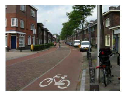
In this example, from Utrecht, NL, space for cycle lanes of adequate width is achieved through making the street one-way for motor vehicles
