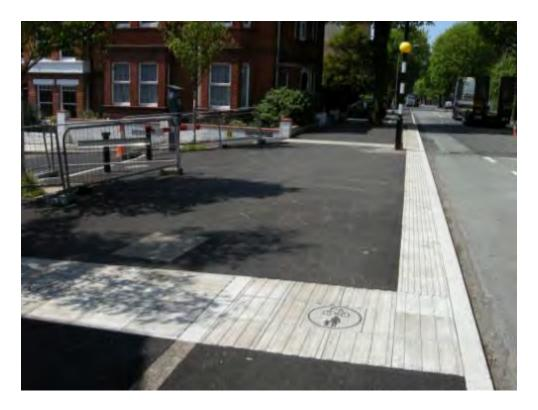
Filtered permeability where a residential side road meets a cycle track on a main road (under construction on Old Shoreham Road, Brighton). Not only does this arrangement remove rat-running on the residential street, it also eliminates turning conflicts across the cycle track.
