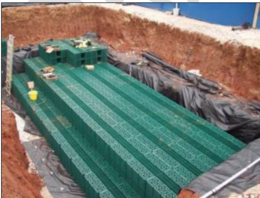
Figure 60. Underground Cellular Storage Tank
