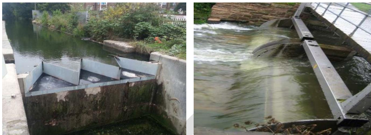
Figure 57. Crenulated and Tilting Weir Structures
