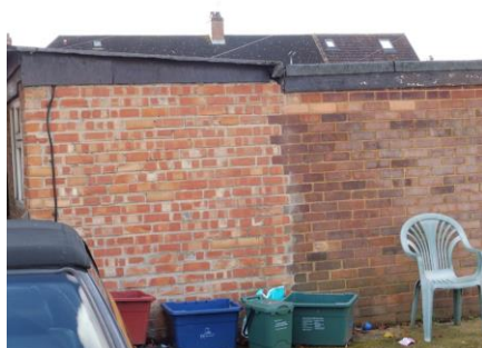
Out building of 48 Beech Avenue toothed into north garage side wall.
