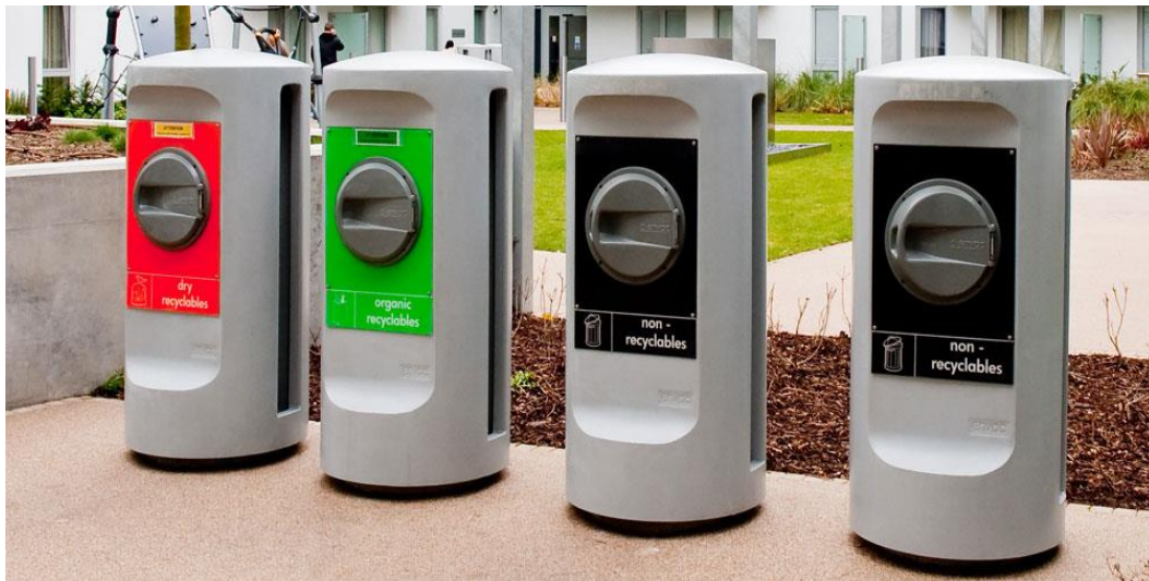
Figure B 2: Waste inlets at the courtyard of the Wembley City development
