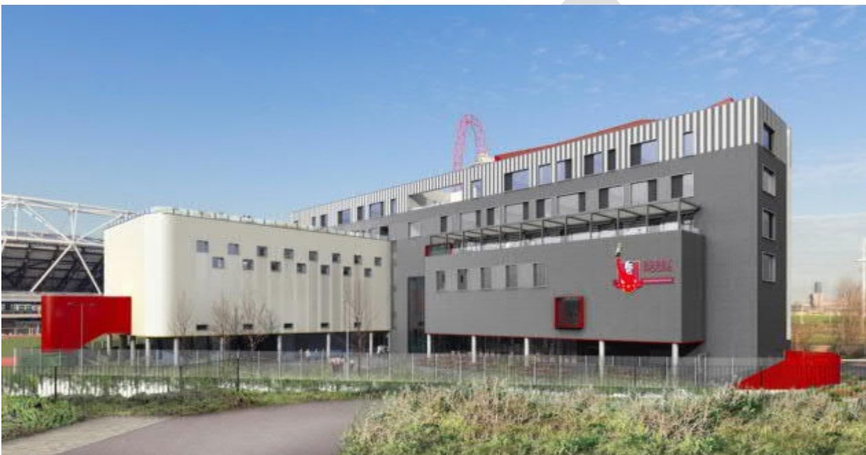
Figure E.3. Bobby Moore Academy – Secondary School
