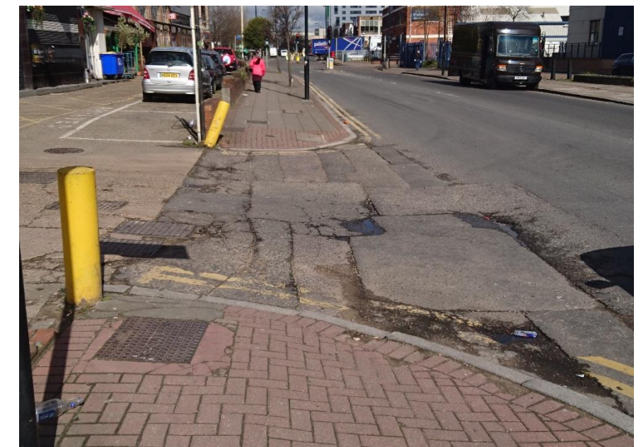
Figure 4-18: Poor surface quality at vehicle crossover (L23)
