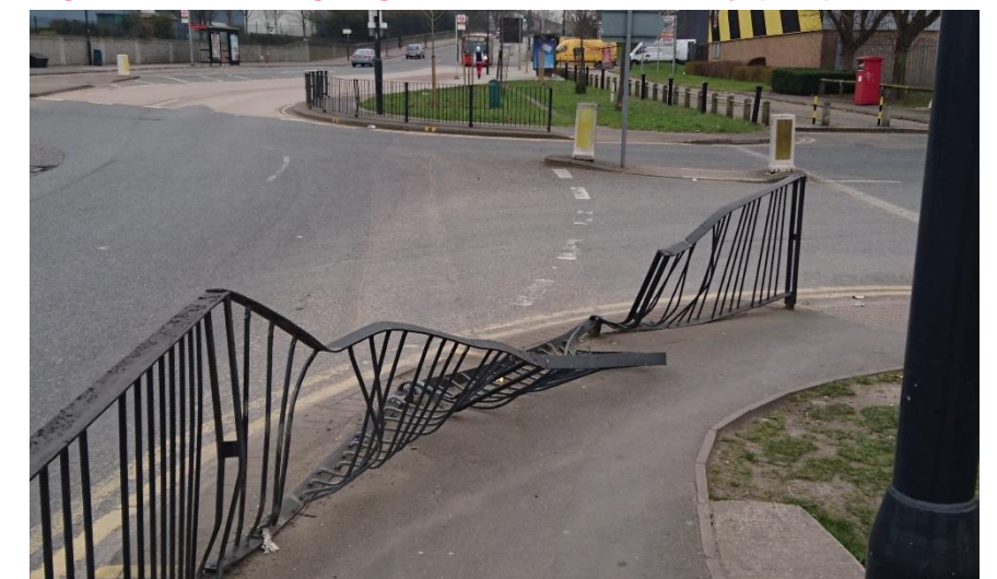
Figure 4-37: Damaged guard rail in the footway (C58)
