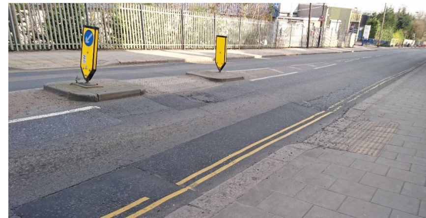
Figure 4-35: Carriageway damage at crossing (C22)
