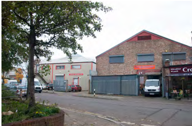
Existing condition Entrances for servicing, office access, visitors and food and beverage uses are intermixed along a street.
