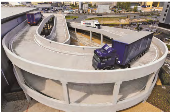
Multi-storey warehousing (X2, Heathrow) Vehicles access service yards on upper storeys via vehicle ramp
