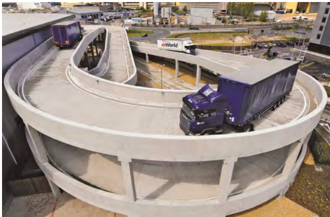
Multi-storey warehousing (X2, Heathrow)
