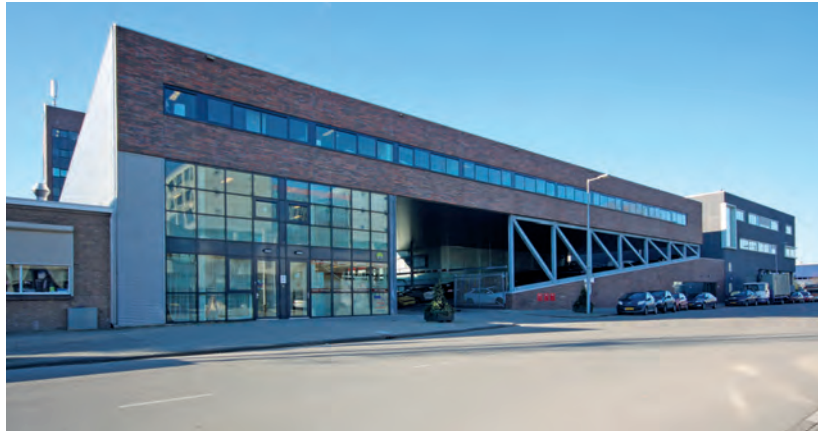
Kaap Nord Offices above workshops, with service access
