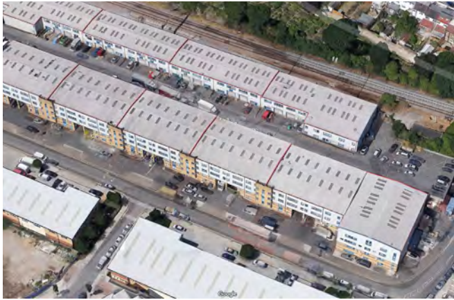
Stacked Industry (Theydon Road, Hackney) Smaller industrial units are stacked above larger units through the provision of a ramp serving multiple units at first floor level.
