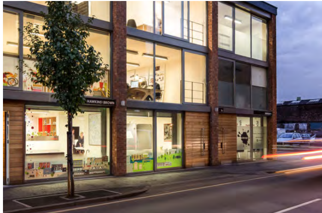
Street presence, Manchester Workspace with strong positive street presence.
