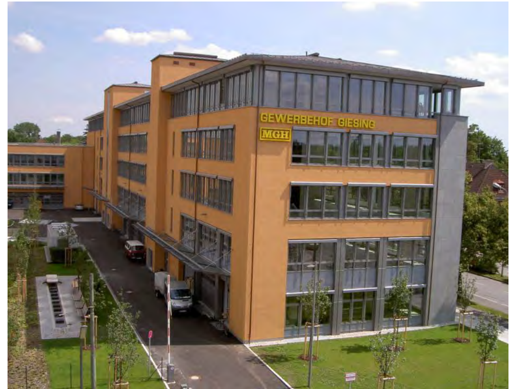
High density workspace, Munich
