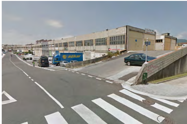
Multi-storey industry (Belasco Building, Irun) Ramps provide access for service vehicles, enabling industrial space to be accommodated on first floor.
