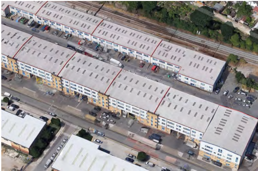
Stacked Industry (Theydon Road, Hackney) Smaller industrial units are stacked above larger units through the provision of a ramp serving multiple units at first floor level.
