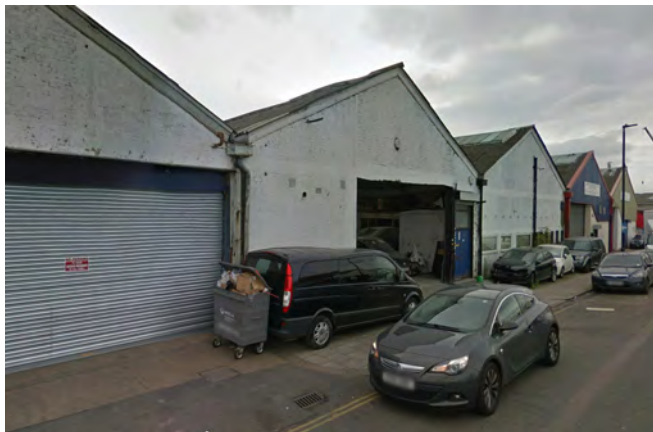
Existing condition Small industrial units have individual, separate loading access within minimal external space for loading.
