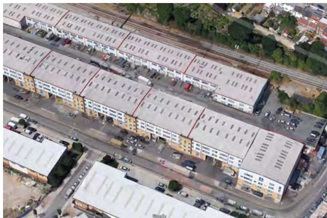
Multi-storey industry, Theydon Road, Hackney
