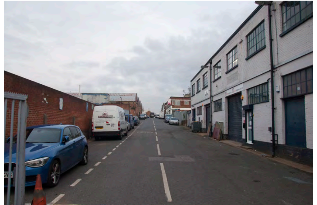
Sunbeam Road Southern edge of site on Sunbeam Road
