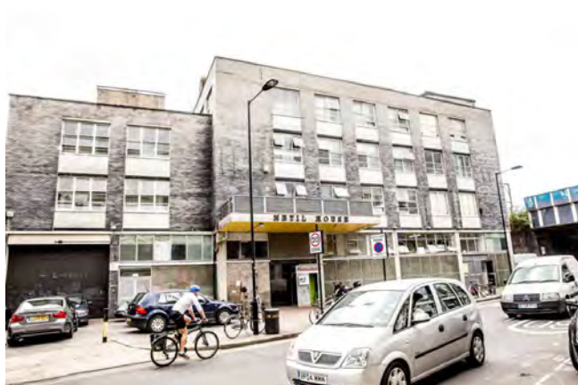
Intensive Workspace (Netil House, Hackney) Good transport accessibility presents the opportunity for large buildings offering intensive mix of workspace
