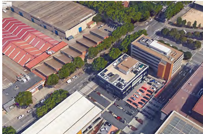
Create distinct street types (Poligon Industrial del Beson, Barcelona) Distinguishing between servicing and pedestrian friendly streets creates a more articulated public realm.
