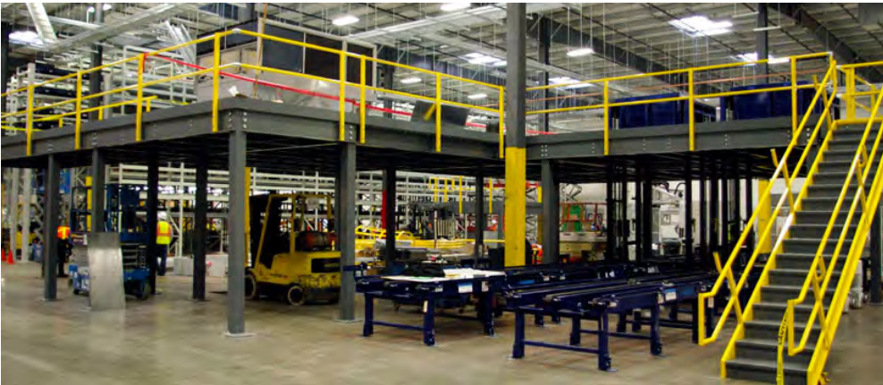
Mezzanine Mezzanine levels provide significant increase in warehouse spaces.
