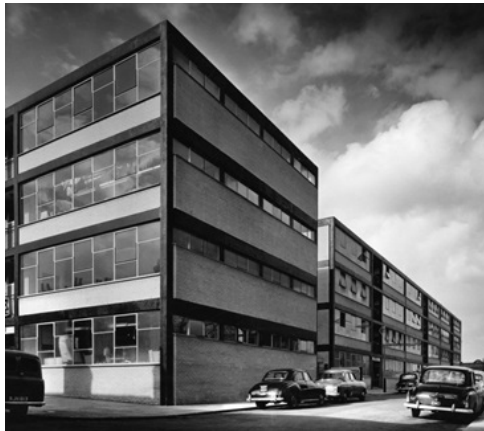
Flatted Factories (London) Workspace can be located above workshops with access from yard space
