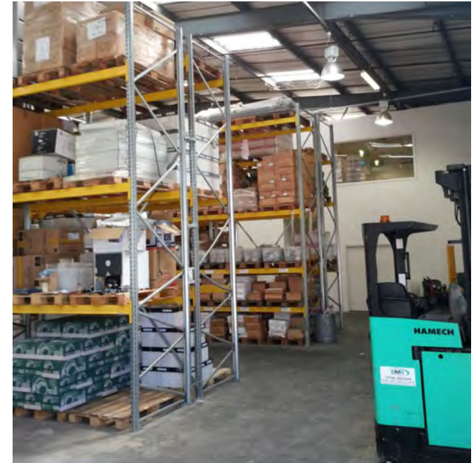
Existing building The existing warehouse space is used for storage.
