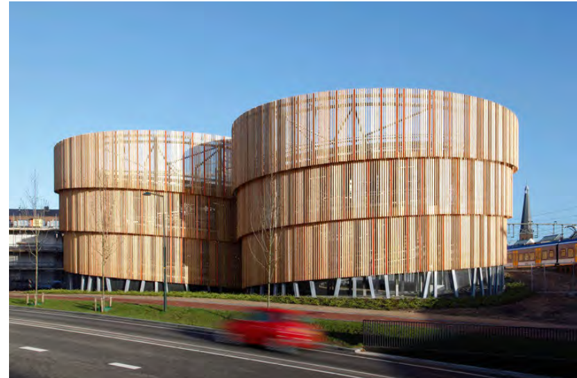
Cladding (P+R Car Park, Zutphen)
