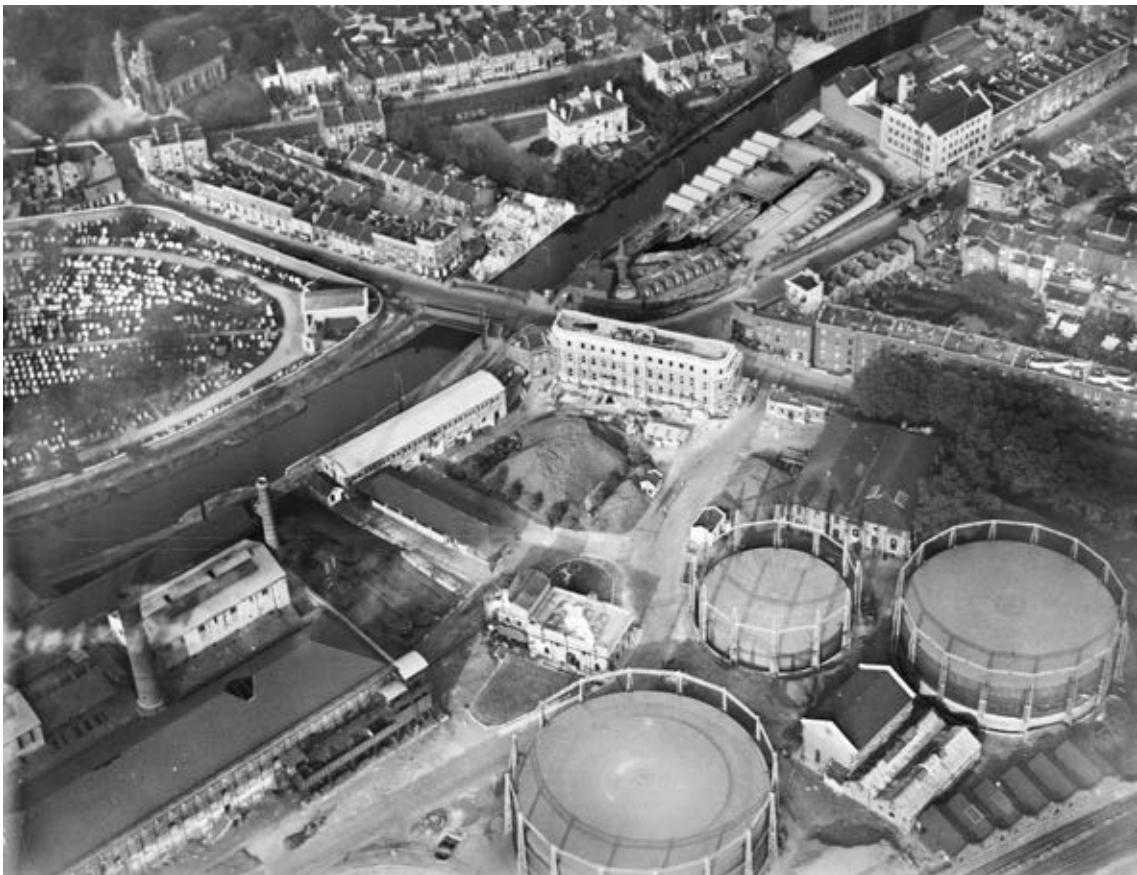
Figure 9: This oblique aerial photograph of 1928, taken from the west-south west, shows part of the Kensal Green Gas Works including Canalside House under construction and coal barges mooring at No. 1 Basin. Beyond is Ladbroke Grove, the Nonconformist Mortuary Chapel of Kensal Green Cemetery, the Grand Union Canal, Corporation Yard, St John's Church and the Regency villa known as Kensal House. The Great Western main line is at the bottom right hand corner. Compare fig. 7, probable taken on the same Aerofilms sortie. EPW024753 © English Heritage. Aerofilms collection.
