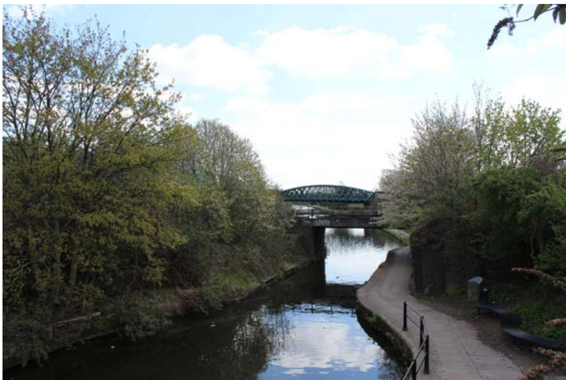
Figure 4: The Grand Union Canal viewed from the Old Oak Lane overbridge. In the foreground is a winding hole, a wider area used for turning a canal boat. 'View corridors' are framed by vegetation and bridges (P6846002).
