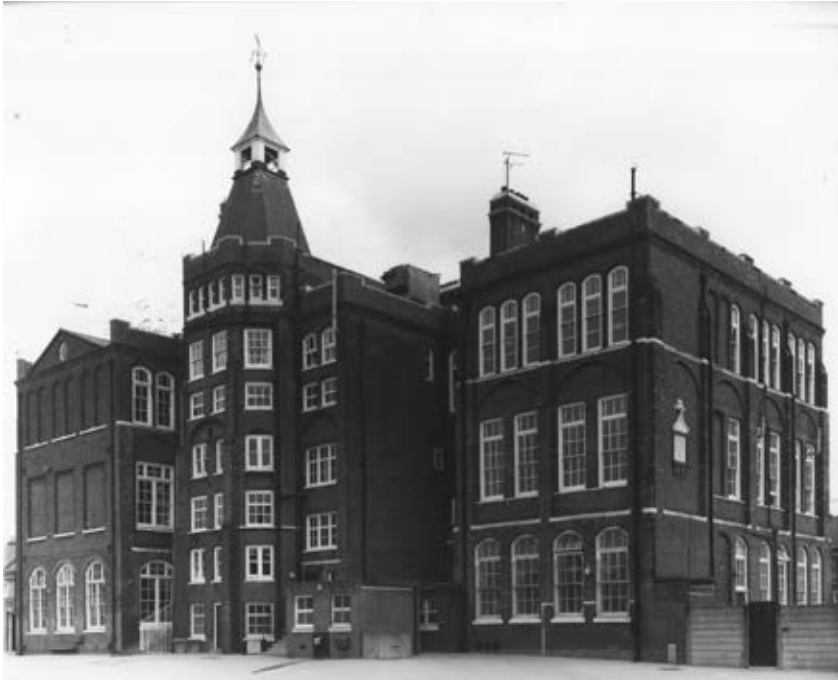
Figure 53: A 1977 photograph of Kenmont Primary School (English Heritage London Region photographic collection, box 306, ref. 77/8423).
