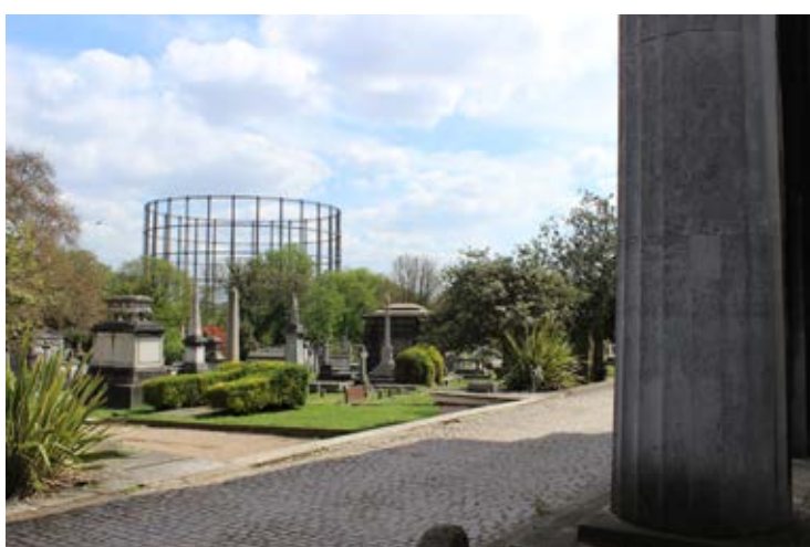
Figure 41: The gasholder forms an element of the setting of Kensal Green Cemetery. South eastern view from the steps of the Anglican Chapel (P6846022).
