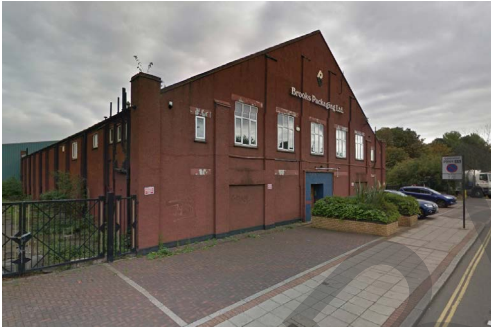
View to south Existing warehouse on North Acton Road
