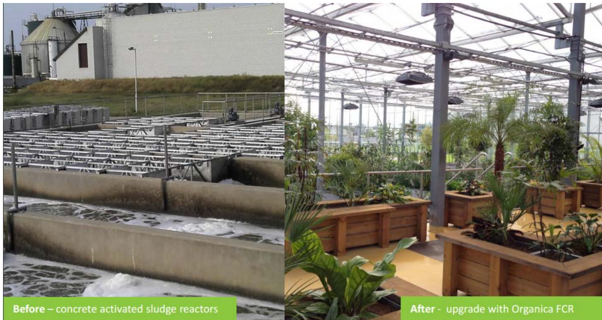
Figure 5-14 - Organica's 80,000m 3 plant in South Pest (source: Organicawater.com)
