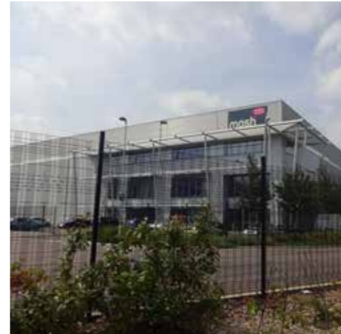
Large modern warehouse unit west of Rainsford Road, buildings step back from road
