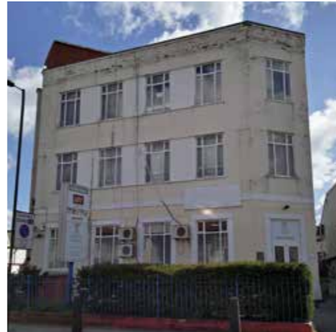
Three-storey brick building fronting onto corner of Everitt Road and North Acton Road
