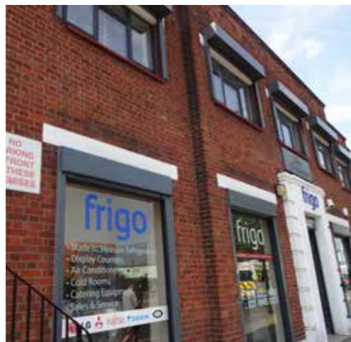
184 Acton Lane makes a positive contribution to the townscape and is one of the earliest buildings in the area, occupied as a utilitas works in 1930s onwards
