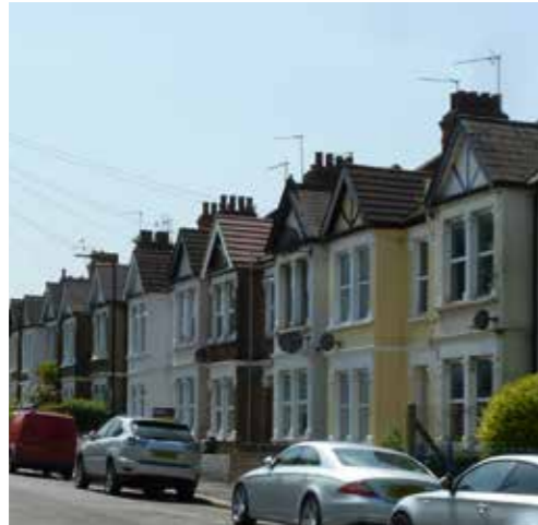
Midland Terrace, a group of late Victorian terraces with two storey flat fronted bay windows with flat columns, and scalloped decorative plasterwork
