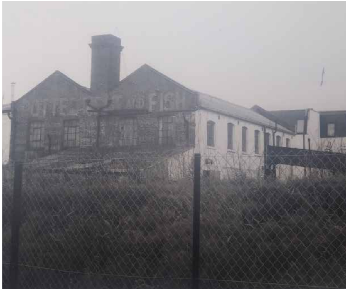
1980 photograph of the back of no. 3 Hythe Road from Salter Street, now demolished Reproduced with the permission of Hammersmith and Fulham archives
