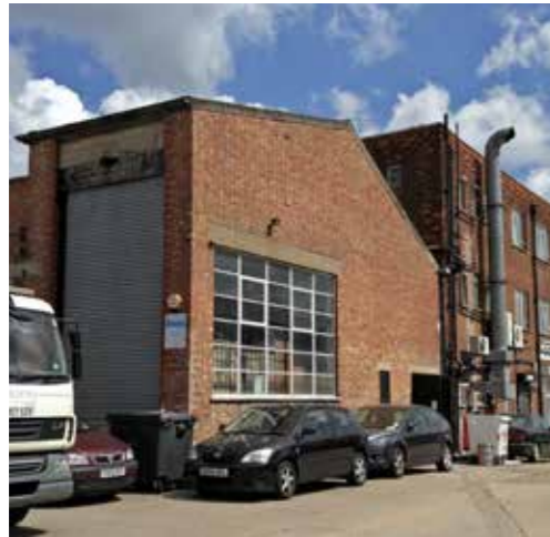
Industrial buildings in red brick front Trading Estate Road
