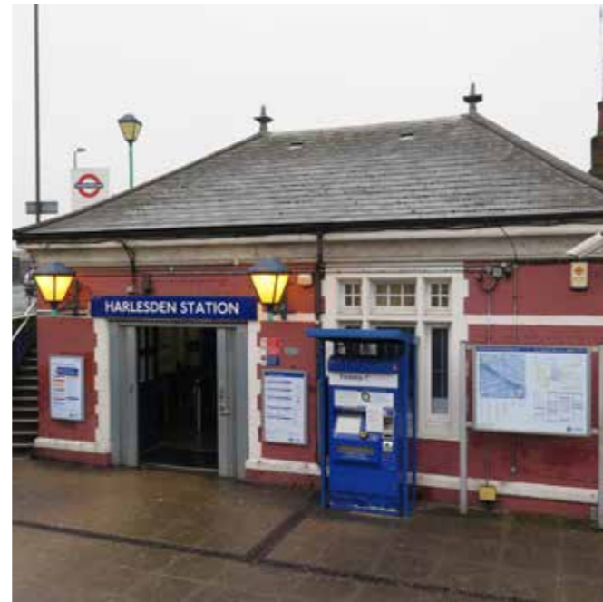
18. Harlesden station, Acton Lane NW10 8UP
