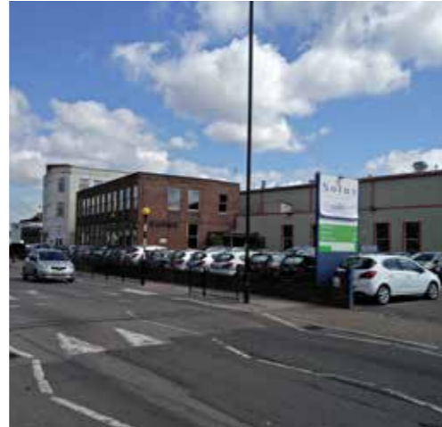
Outdoor car parking onto North Acton Road creates an uneven edge and disjointed edge along the road
