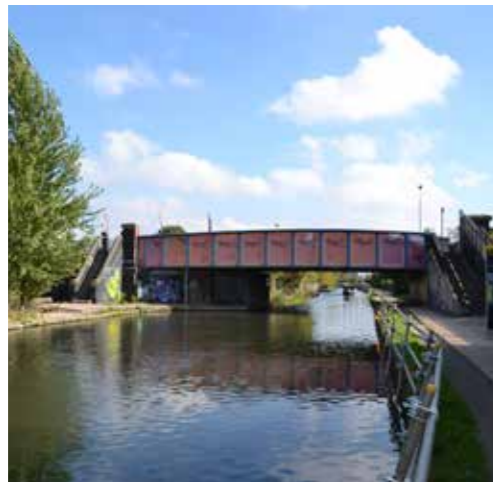
Mitre Bridge, recommended for local listing
