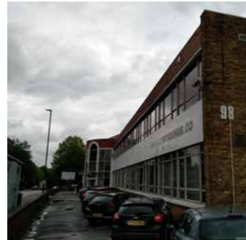
View of building at north of site
