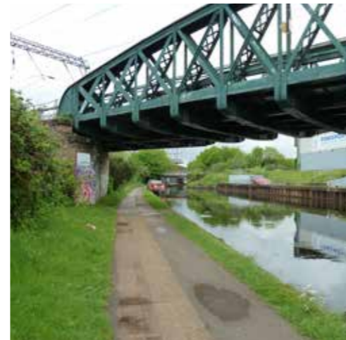
View looking west, the Kew Curve Grand Canal rail bridge crosses the canal near Powerday, recommended for local listing
