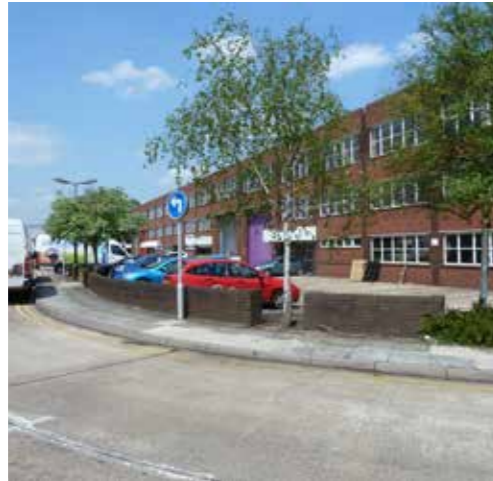
View north-west along Concord Road. 1960s three storey industrial units set back from the road. Recent tree-planting gives greenery to a predominantly industrial landscape.
