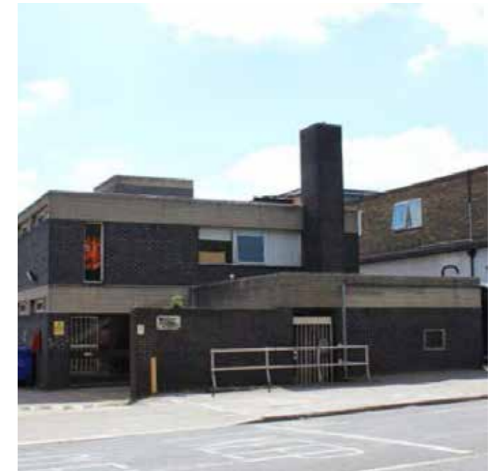
8. Network Rail's Willesden Junction Maintenance Depot, Old Oak Lane, NW10 6EJ
