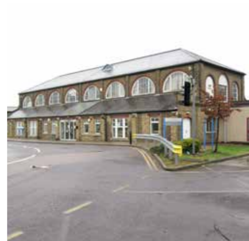
The Old Refectory on Central Way, two storeys with stock brick and red brick dressings with a hipped slate roof
