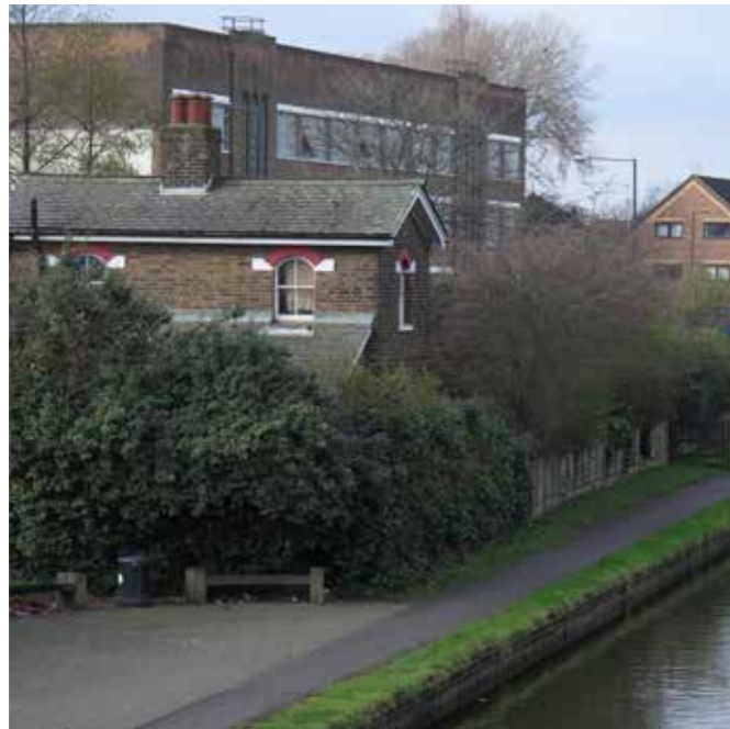
5. Canal Cottage by Grand Union Canal Twyford Abbey Road, NW10 7DE
