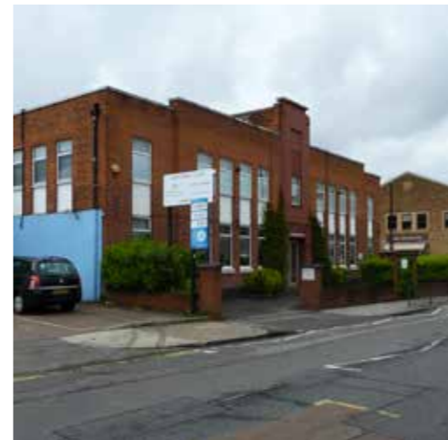
Former premises of John Compton Organ Makers, Chase Road. Rebuilt after bomb damage in the Second World War.
