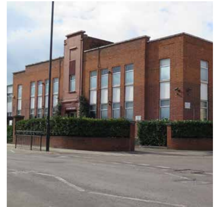
16. Former Compton works, Chase Road NW10 6HZ
