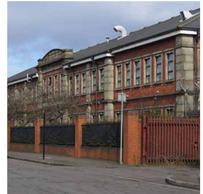
4. Metal Refinery, Bashley Road NW10 6SN
