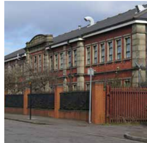
The Metal Refinery building, Bashley Road
