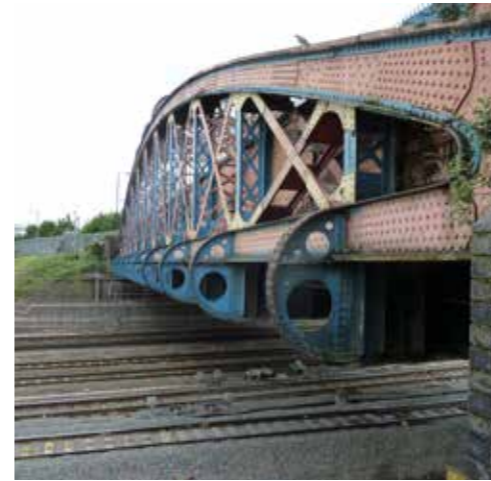
Scrubs Lane Overbridge, carrying Scrubs Lane over the Great Western main line and reconstructed in 1905, recommended for local listing
