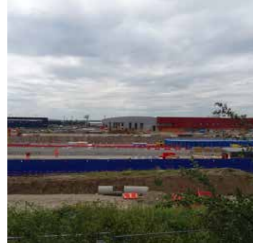
View looking south at the construction site of the new Crossrail depot for the Bombardier trains, which can be seen in the background
