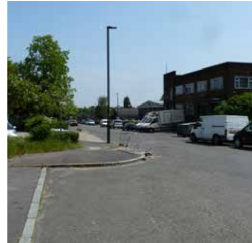
The area is dominated by hard concrete surfaces and there is negligible greenery
