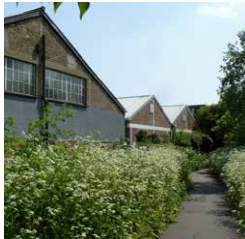
A footpath remains to the west of the character area which follows the former Mason's Green Lane, linking Park Royal tube station with the Hanger Hill Estate, a residential area to the south
