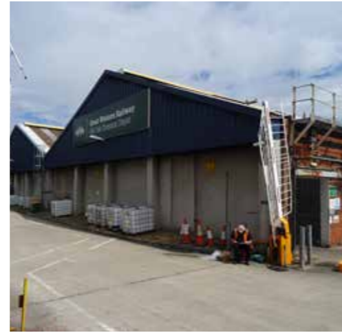
Existing Great Western Railway Old Oak Common Depot, one of the few remaining buildings from the early 1900s, although heavily altered
