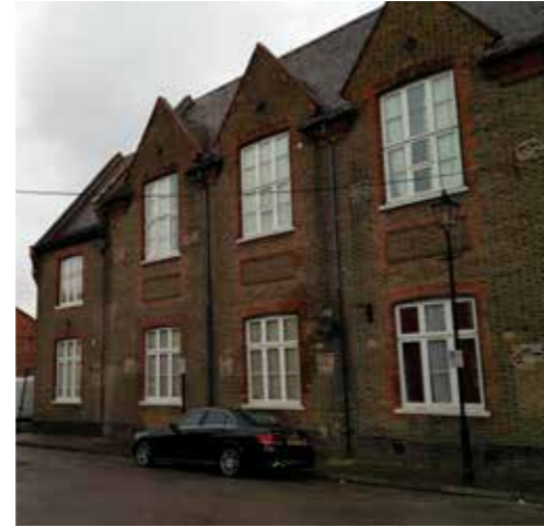
Former Railway Institute is a positive contributor to the townscape
