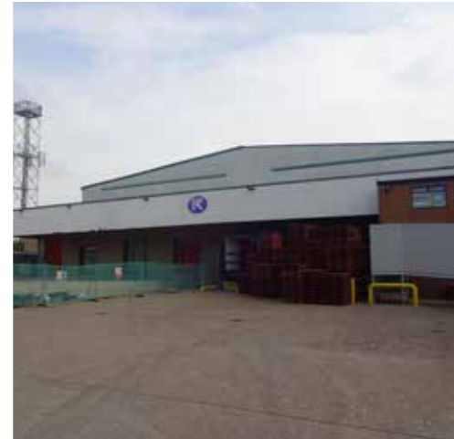
Warehouse building on Elveden Road at junction with Elveden Place, used by Kolak Foods Ltd.
