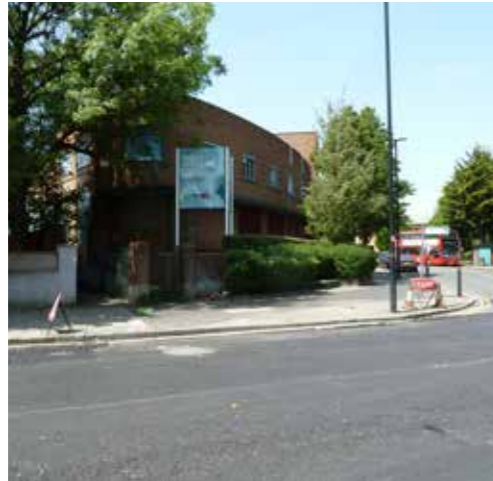
Entrance to Brunel Road from Old Oak Common Lane
