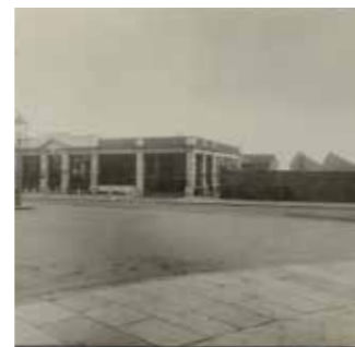
pre 1925 photo of Dubilier Condenser Co. building fronting Victoria Road with factory in background Reproduced with permission of the Ealing Local History Centre
