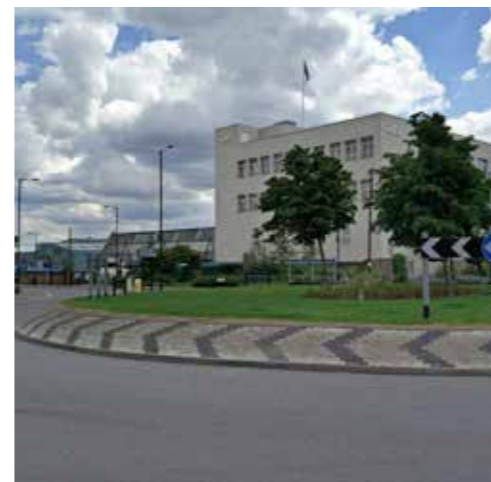
View of HMR on corner of west side of Cumberland Avenue and Rainsford Road
