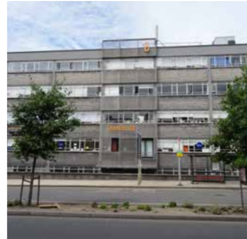
View of Chandelier building, five-storey 1960s building, of positive importance to townscape and suitable for re-use
