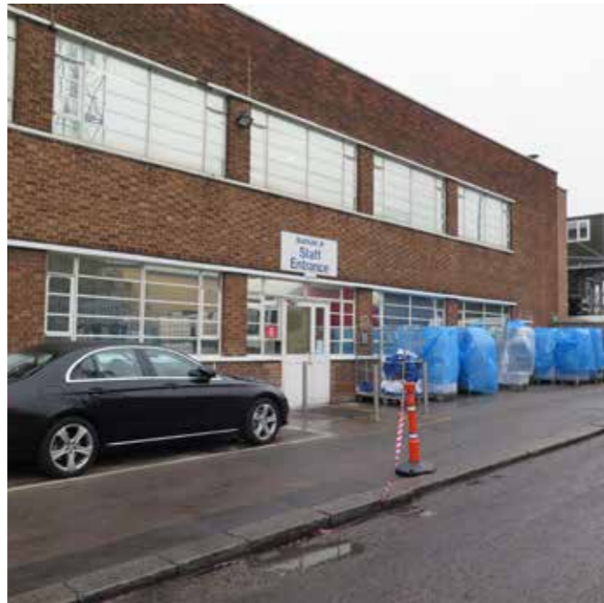
21. 304-306 Elveden Road NW10 7SY
