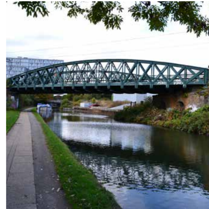
31. Kew Curve Grand Canal rail bridge NW10 6EJ
