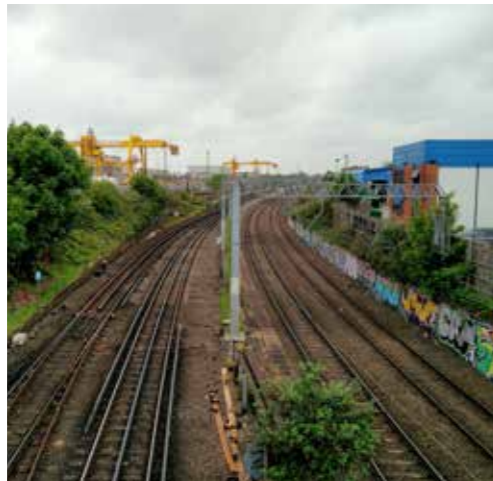
View from Old Oak Lane bridge looking west across the railway lines
