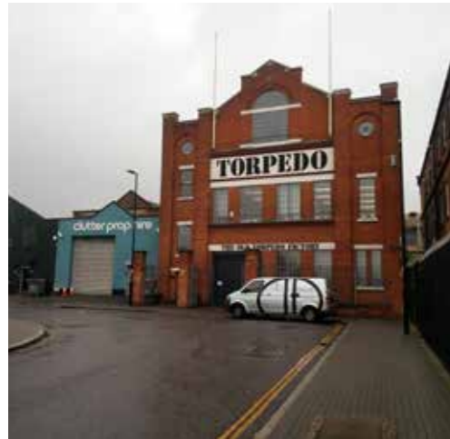
The Old Torpedo Factory building, St. Leonard's Road
