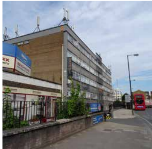
View looking north up Scrubs Lane, with the Chandelier building to the left, built in the 1960s near the site of Ellisland House
