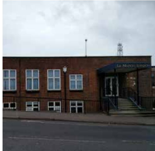
Former Carlsberg building fronting onto Old Oak Lane
