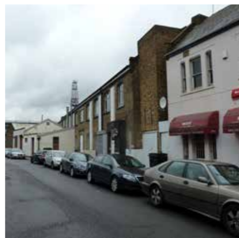
View of Former Engineering Works, 18-19 Hythe Road, proposed locally listed
