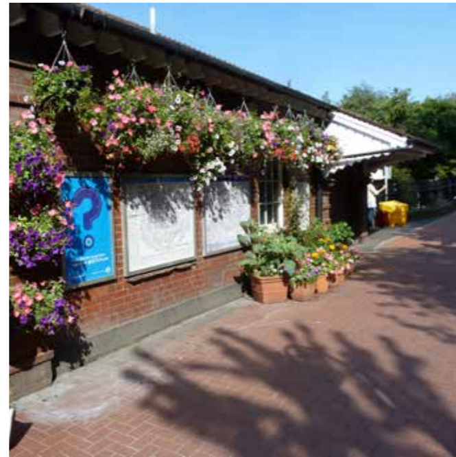
2. North Acton Station, Victoria Road W3 6UP
