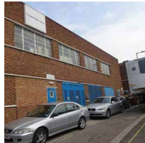
Flat-roofed red-brick building with little active frontage with road
