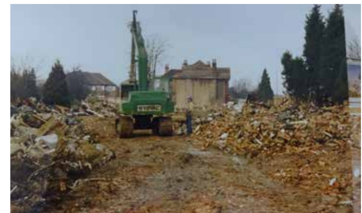
A40 widening scheme led to the demolition of 43-75 Western Avenue, 1996 Reproduced with permission of Ealing Local History Centre
