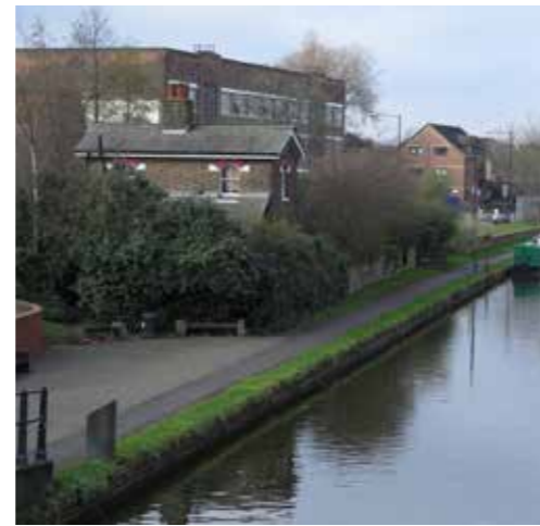
View of Lengthman's cottage, locally listed
