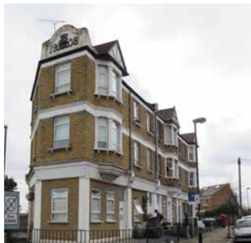
No. 1 Wells House Road was the location of the former Lighthouse that was a permanent feature of the area for many years
