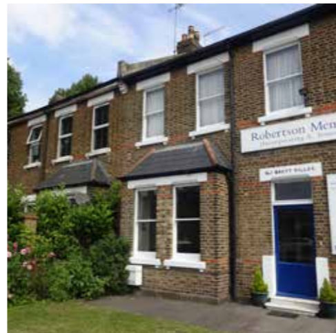
Brett's Villas, a late Victorian symmetrical pair of villas in stock brick with original sash windows and a hipped slate roof
