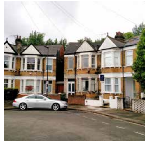
Terraces along Wells House Road
