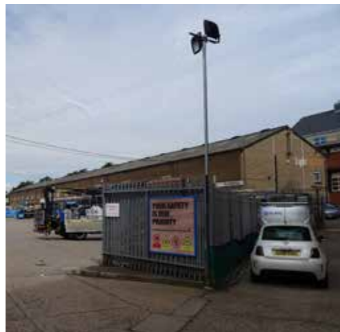
View of Light Factory building to the rear of the Chandelier building, single-storey brick warehouse space
