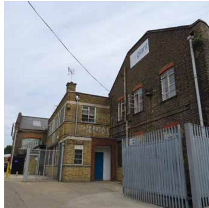
14. Former Gate and Shutter works, south of 1-10 Enterprise Way, NW10 6UN
