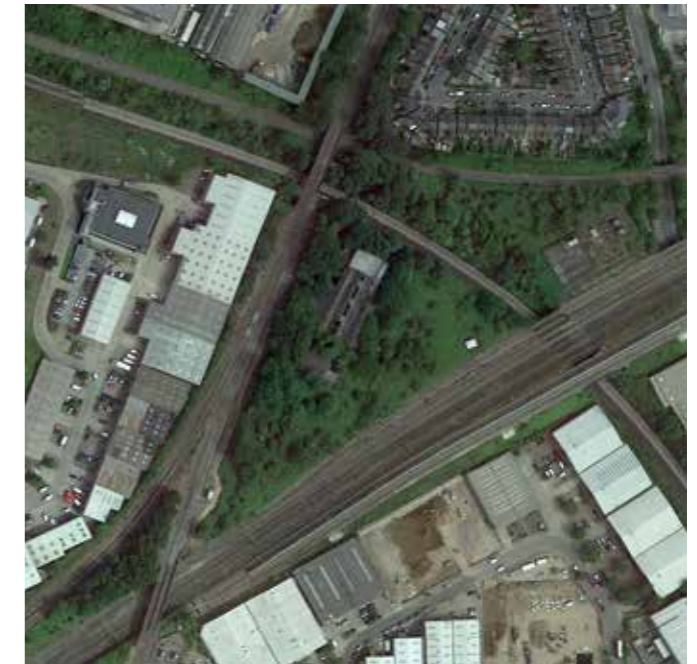
4. Electricity sub-station, south east of Wells House Road
