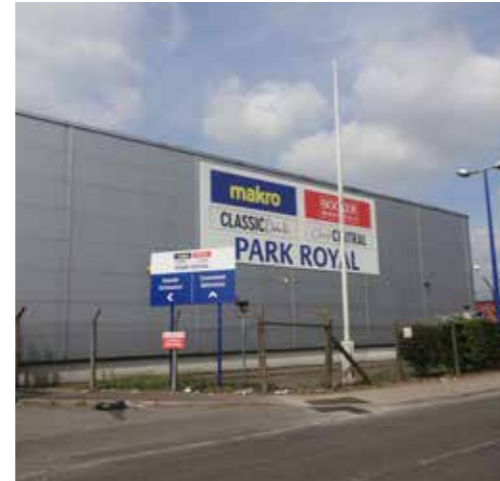
Makro superstore, large free-standing structure with blank frontage
