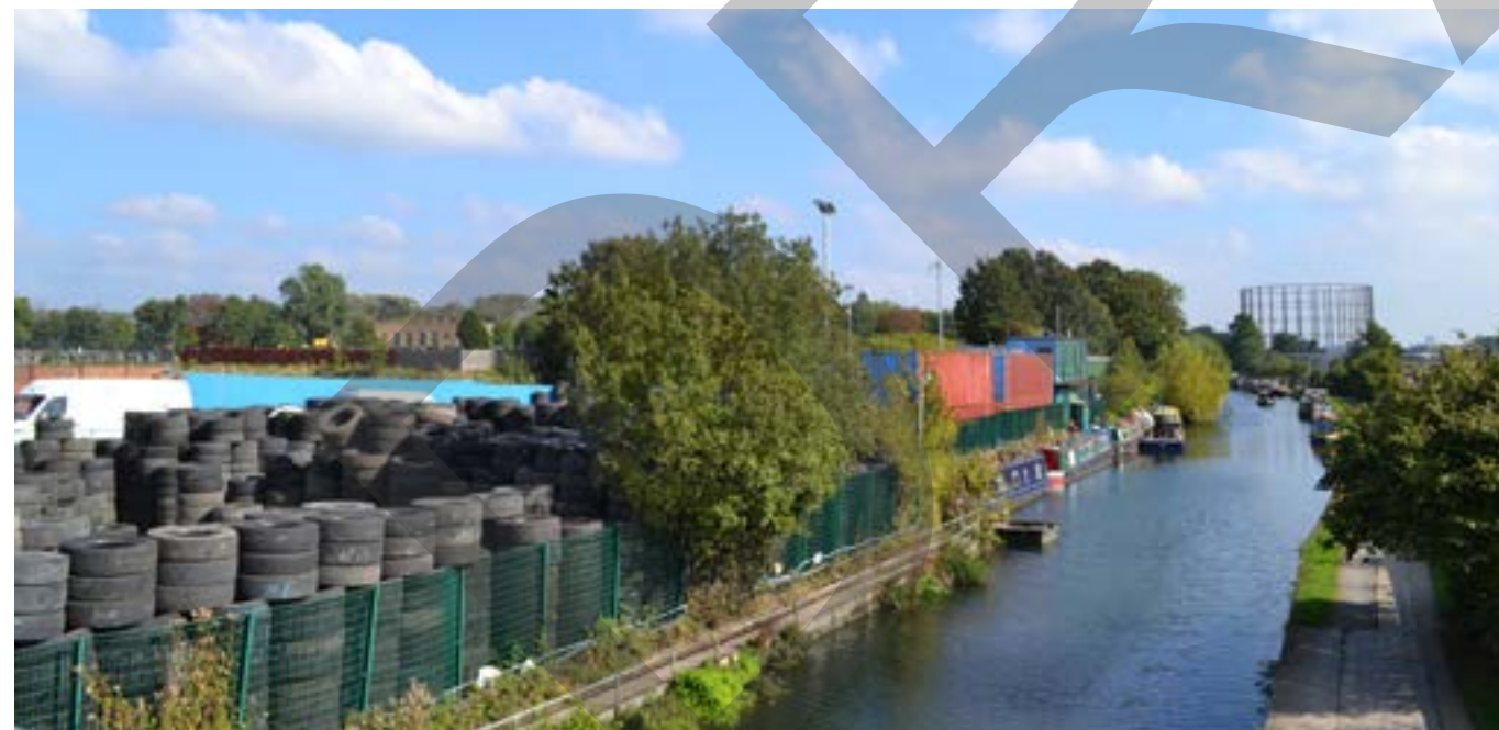
Views towards gasholders
