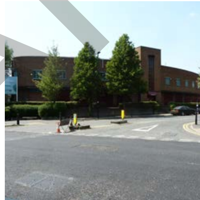
15. 1-17 Farley building, Brunel Road W3 7XR
