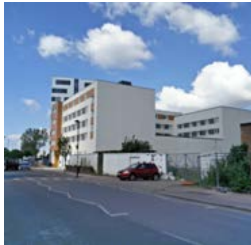
Victoria Care Centre, Acton Lane
