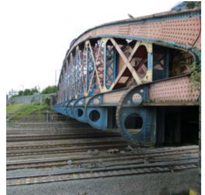
28. Scrubs Lane over bridge NW10 6QE
