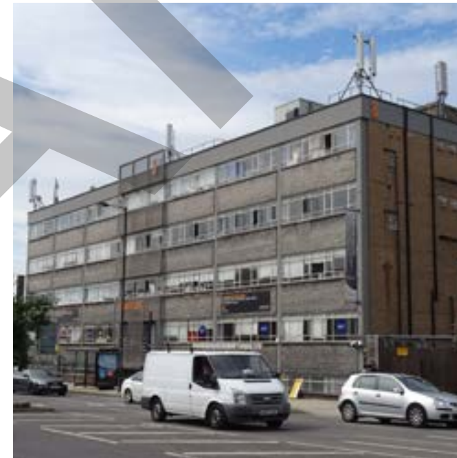
18. Chandelier building, Scrubs Lane NW10 6RB
