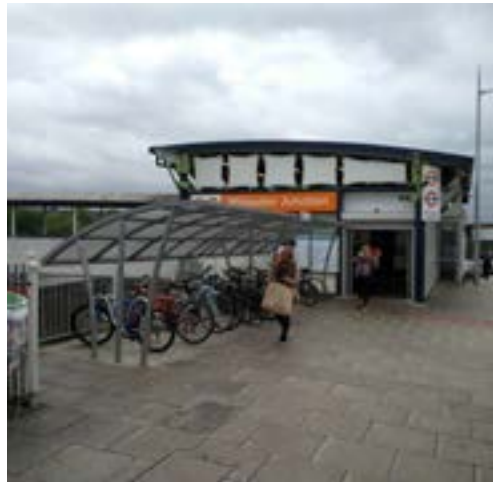
Modern entrance to low-level Willesden Junction station
