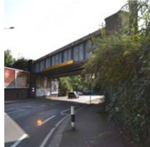
Scrubs Lane underbridge
