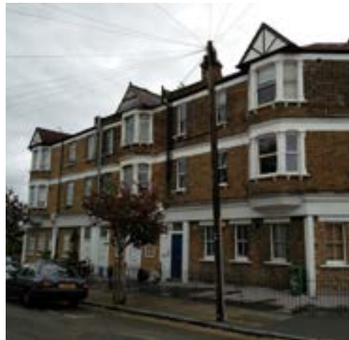
1-5 Wells House Road
