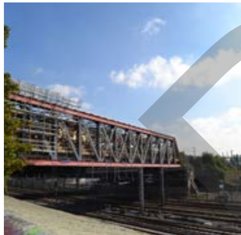
West London Line overbridge, a single-span skew bridge composed of braced steel trusses spans the Great Western main line, c. 1908, recommended for local listing
