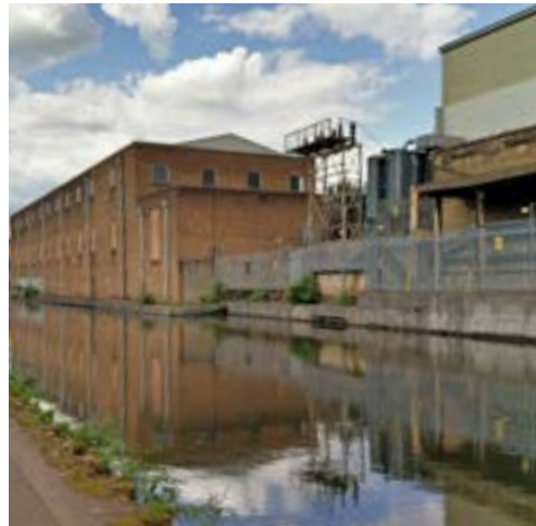
Acton Lane Power Station with dry dock
