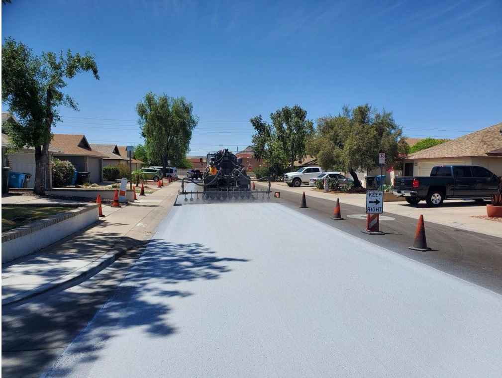
Figure 4. Resurfacing with reflective pavement in Phoenix 7
