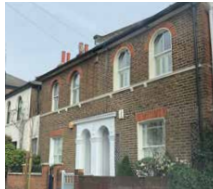
Flat fronted single home terraces
