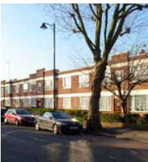
Two-story 1930s block with rows of windows with clear boundary
