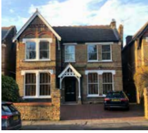
May villas have seen front gardens paved
