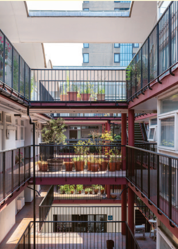
Atrium corridor with natural light makes space for neighbour interaction
