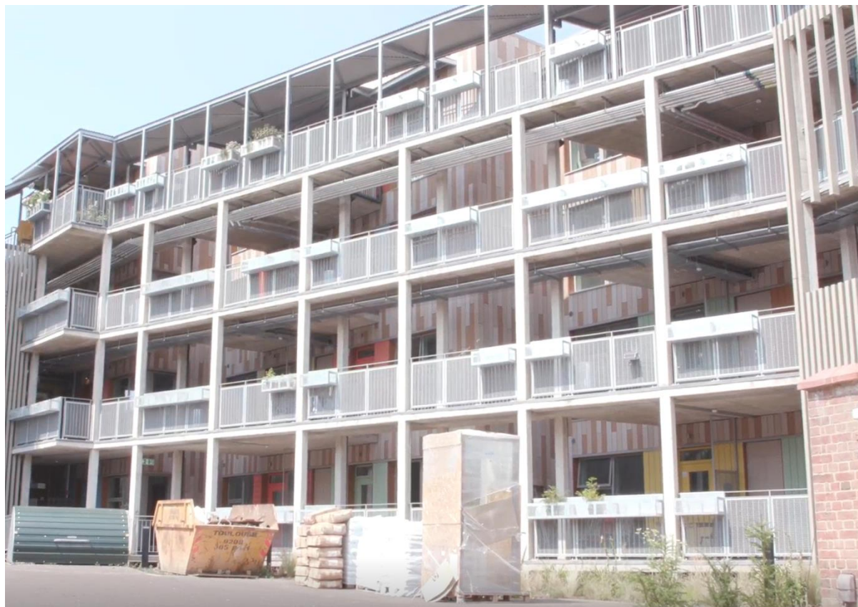
Church Grove (Source: London Assembly)
