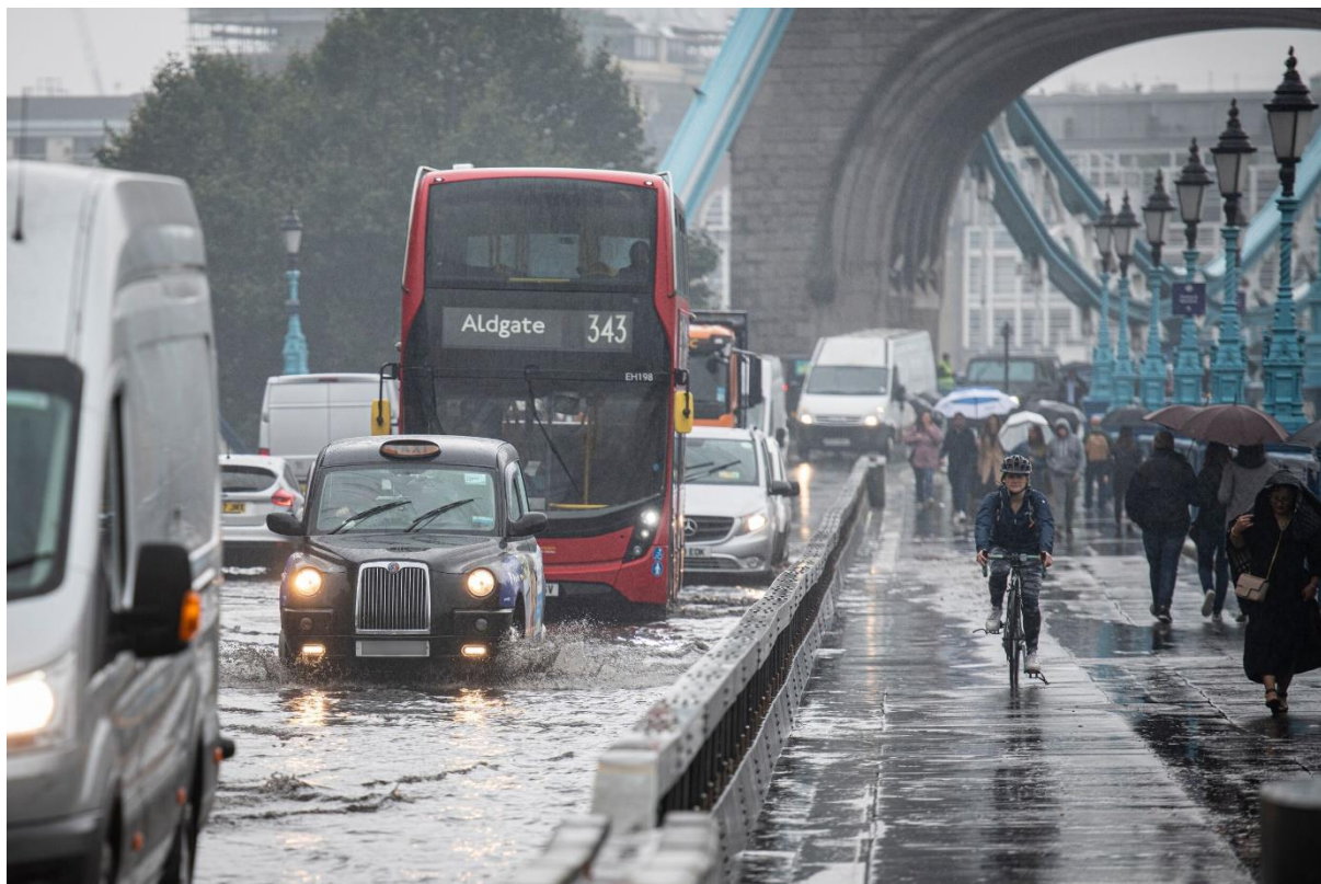
Flooding on Tower Bridge
