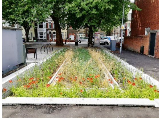
Figure 77: Example of an infiltration basin (Source: Arup).
