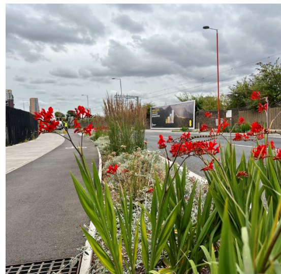
Figure 70: Rain gardens installed in Waltham Forest (Source: Meristem Design)
