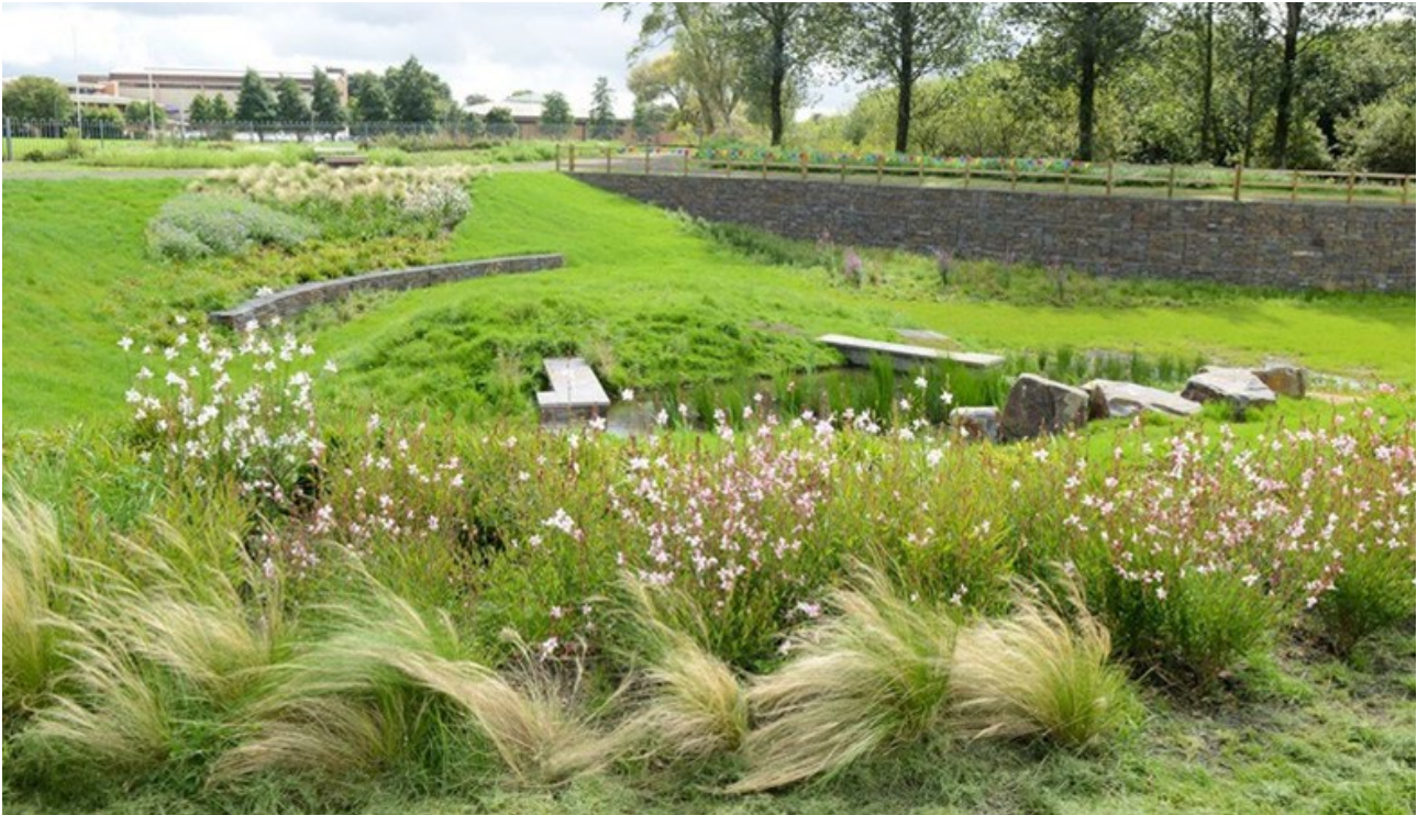
Figure 73: Example of a detention basin at Parkview Terrace, Llanelli (Source: Arup).
