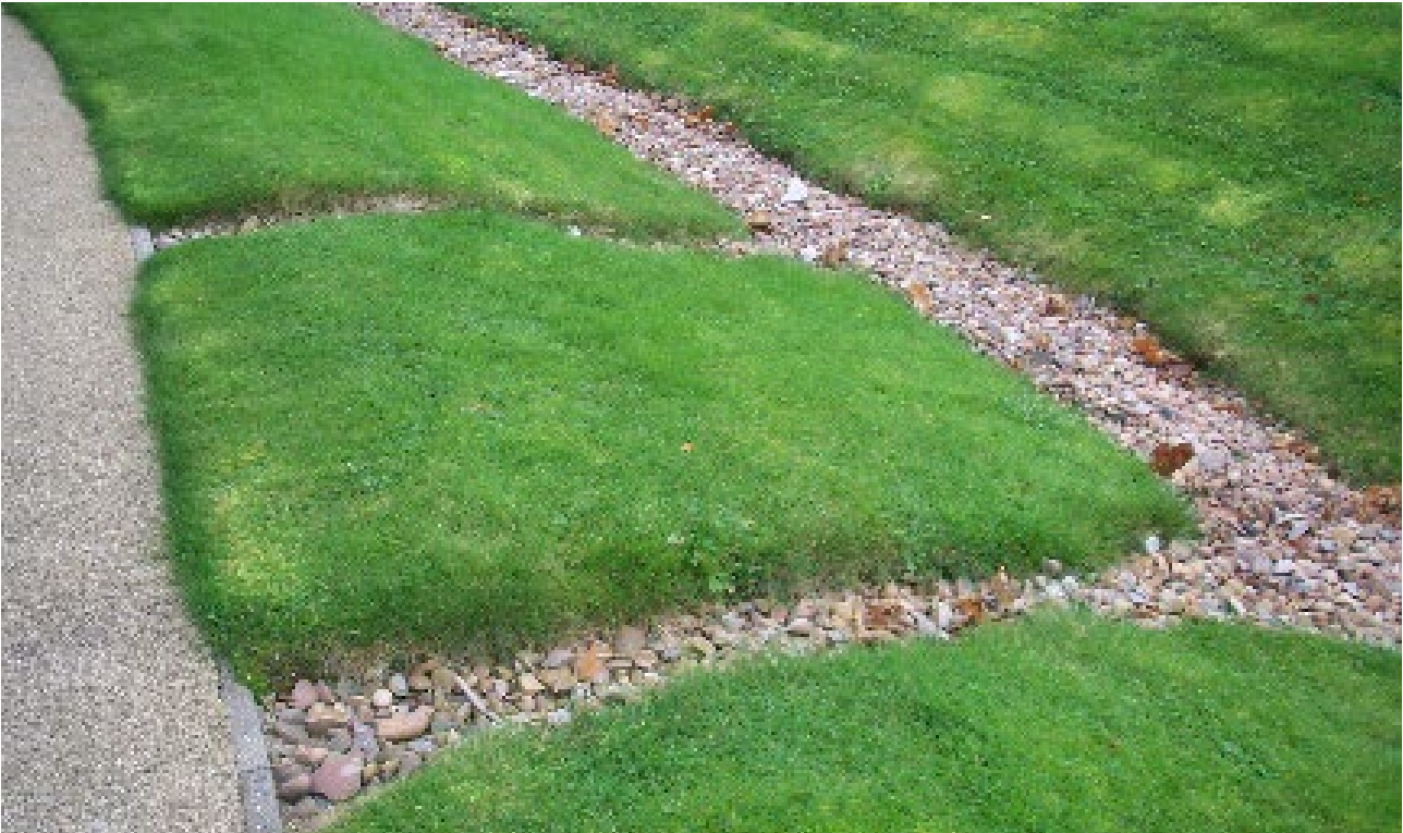
Figure 74: Example of a filter drain (Source: Arup).
