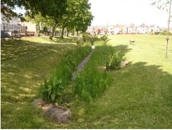
Figure 76: Example of soakaway (Source: Arup).
