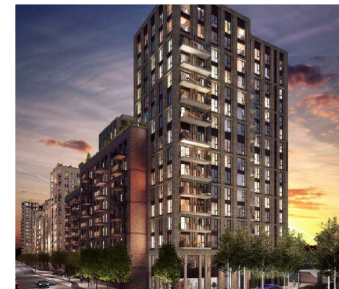
Brunel Street Works
