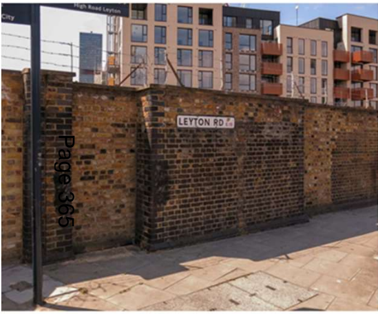
external east facing elevation of the Angel Lane urinals. July 2018
