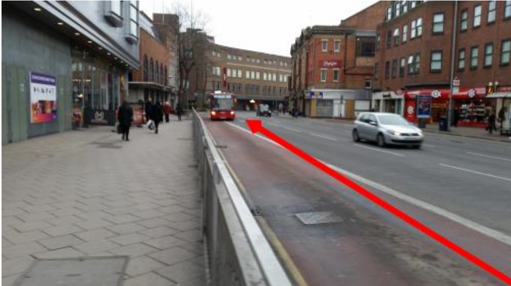
Figure 68 Pipework route along Clarence Street (looking South)
