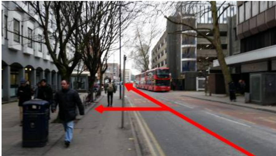
Figure 72 DH pipework along Brook Street and connection to the Old Post Office Development
