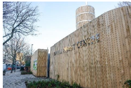
Figure 1. An energy centre. Source: Islington Council
