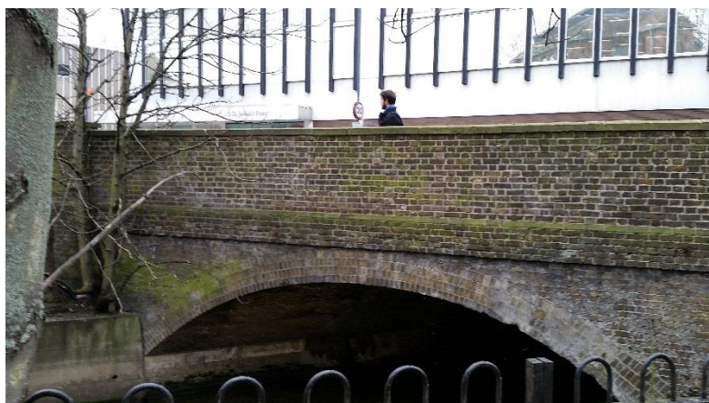
Figure 58 Hogsmill river bridge crossing
