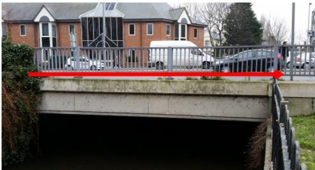
Figure 11 Hogsmill River crossing along Wheatfield Way
