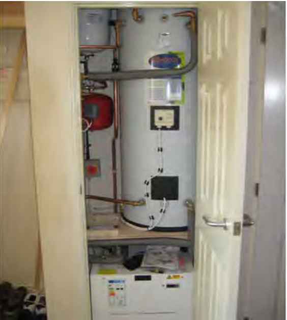
Figure 5.9: Kensa Shoebox individual GSHP installation 24
