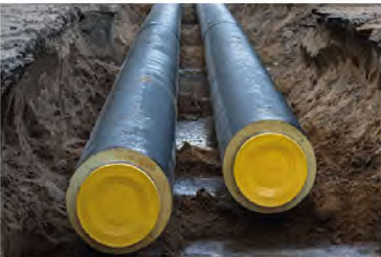
Figure 3.5: Left, example Gas Combined Heat and Power (CHP) engine commonly used in energy centres (Edina). Right, district heating flow and return pipe trench (Enviropipe)
