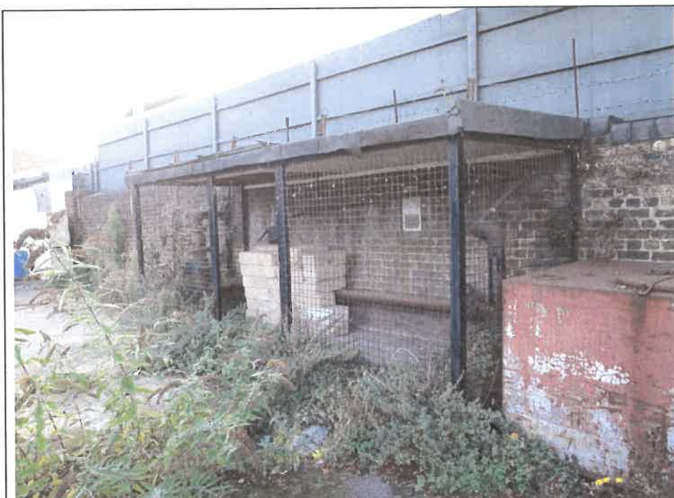
Photo 89: Lean to structure and oil tank
