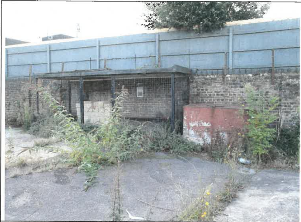
Photo 91: Lean to structure and oil tank
