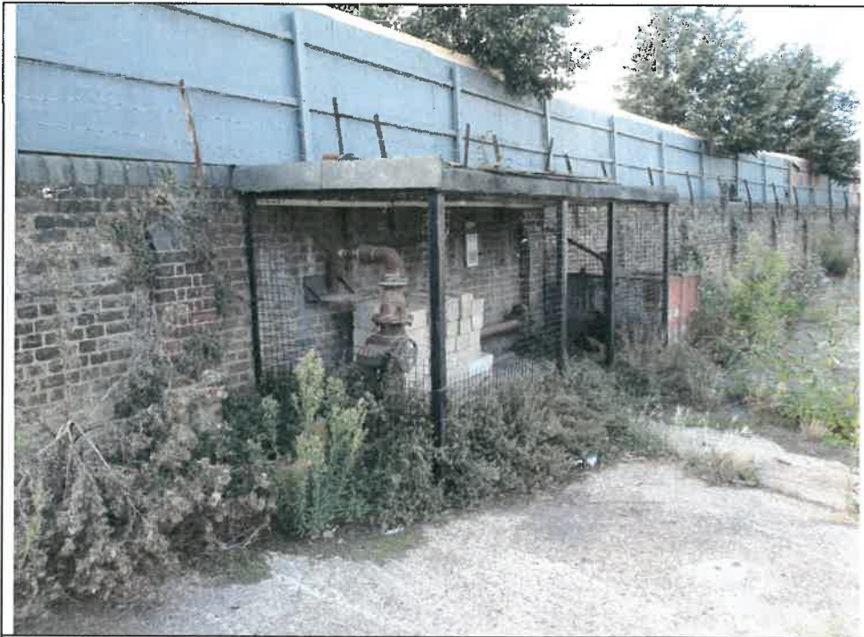
Photo 87: Lean to structure and oil tank
