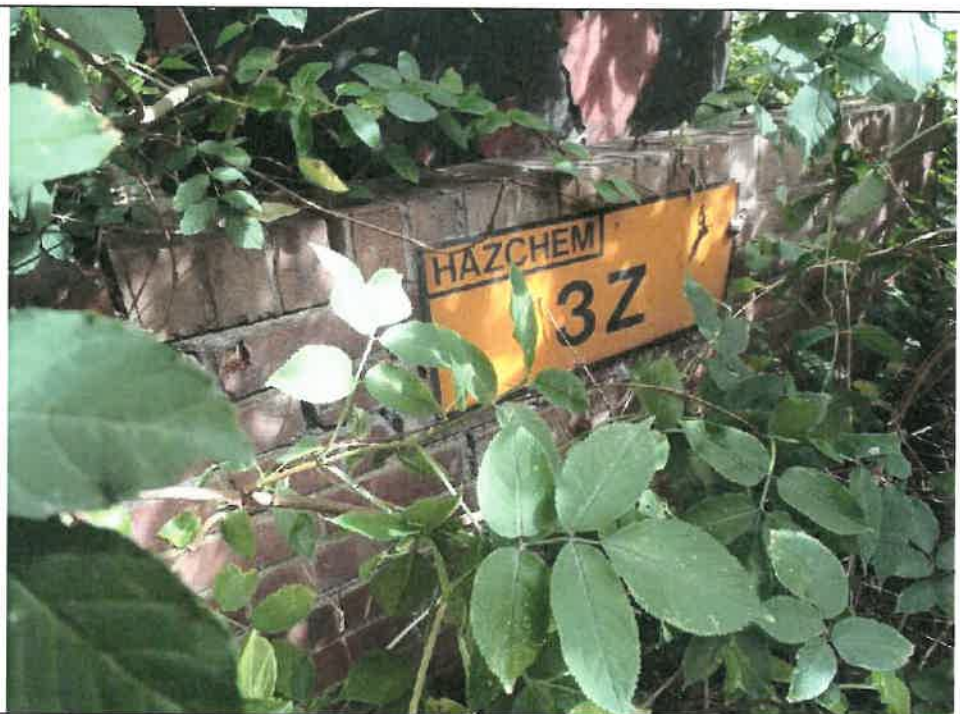
Photo 52: Building 3 – Oil tank to rear
