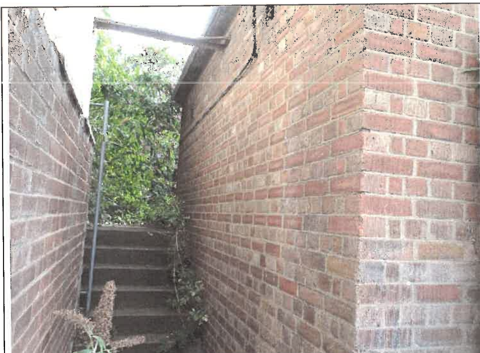
Photo 53: Building 3/4 – Steps to oil tank at rear
