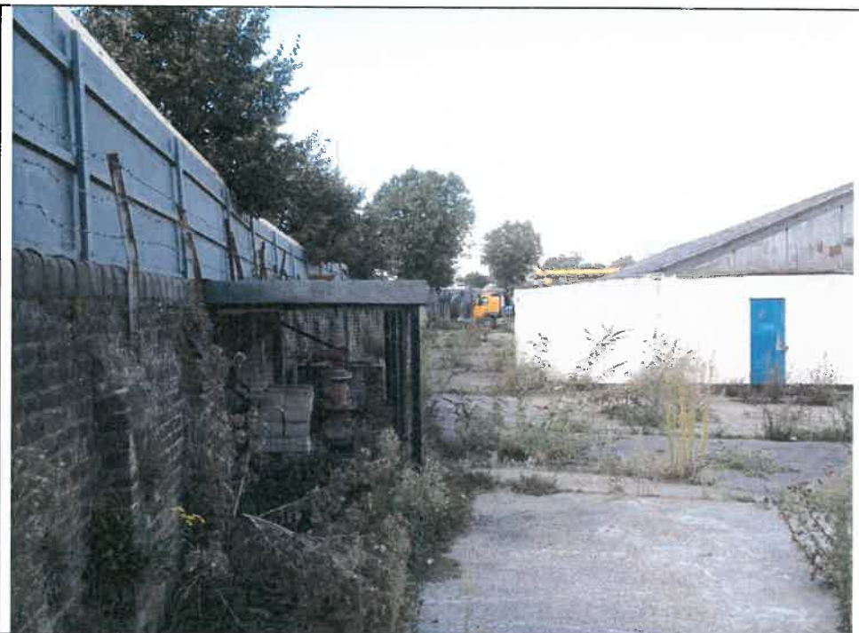
Photo 92: Lean to structure and oil tank
