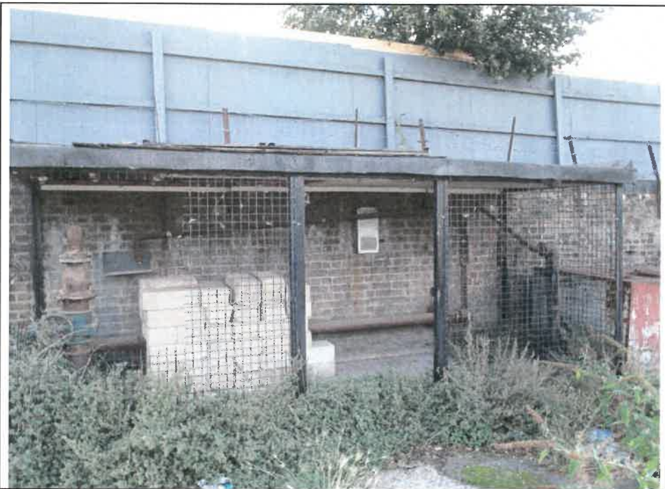
Photo 88: Lean to structure and oil tank
