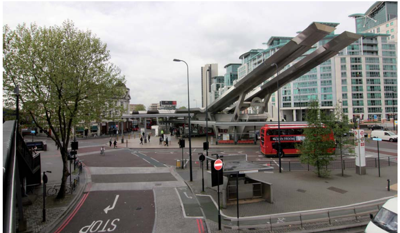
Figure 2.3.2: Fragmented public realm within the gyratory.
