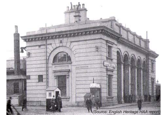
Figure 1.4.1: Nine Elms Station (source: VNEB OAPF)
