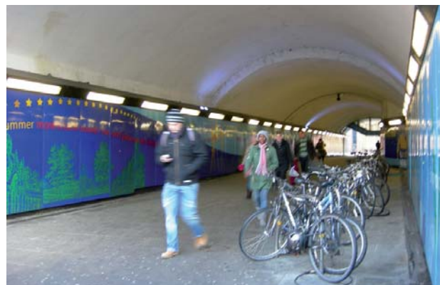
Figure 2.3.4: Pedestrian tunnel through railway viaduct
