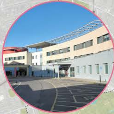
Central Middlesex Hospital
