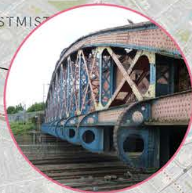
Scrubs Lane Overbridge Mitre Bridge West London Line Overbridge
