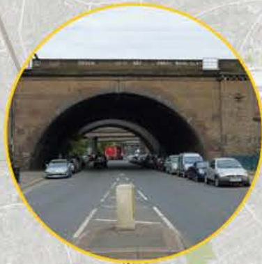
Brent Viaduct (Listed)
