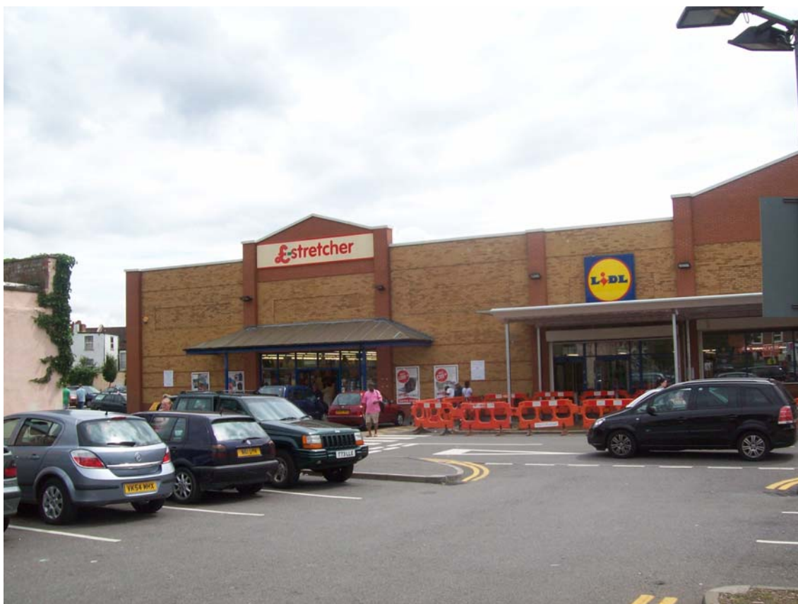
Fig 1: Lidl and Poundstretcher stores to the south of the Uxbridge Road
