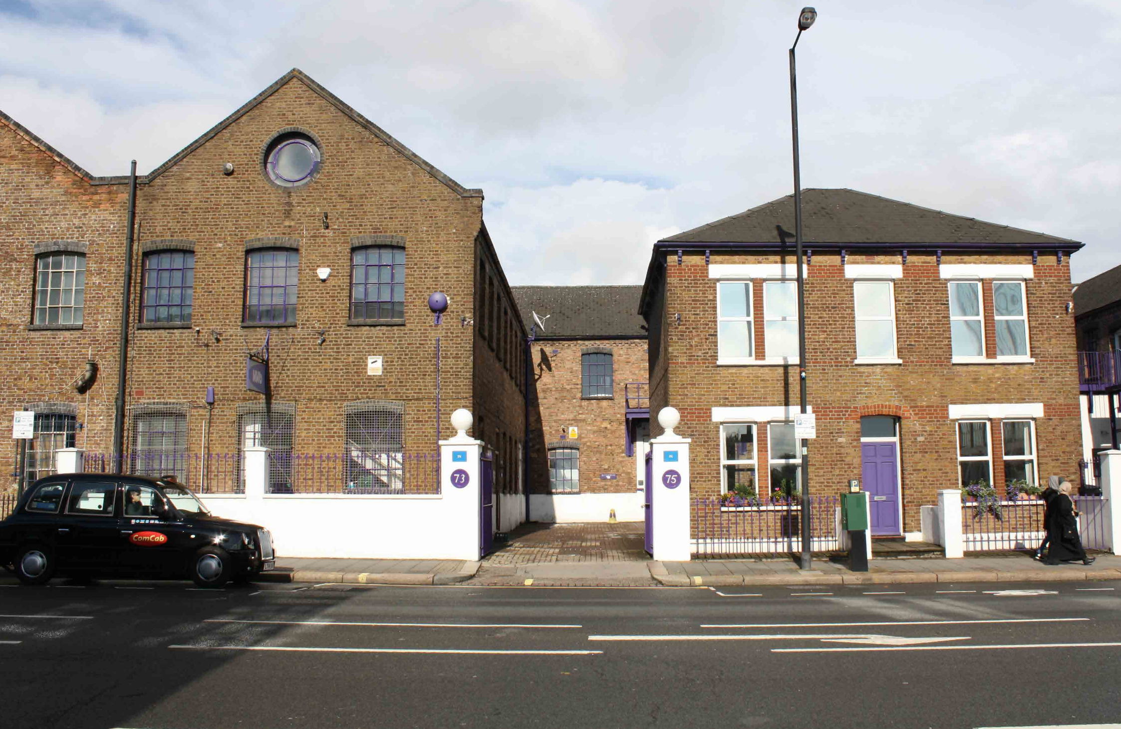
Figure 73: Frontages of proposed Cumberland Park Factory Conservation Area
