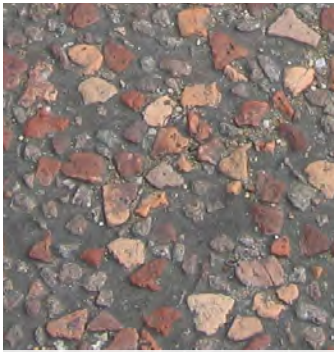
Tarmacadam with granite aggregates
