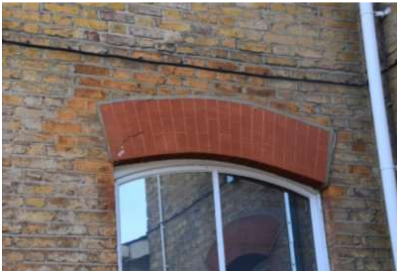
Figure 16: Brick lintel displaying evidence of repair, but also new cracks.
