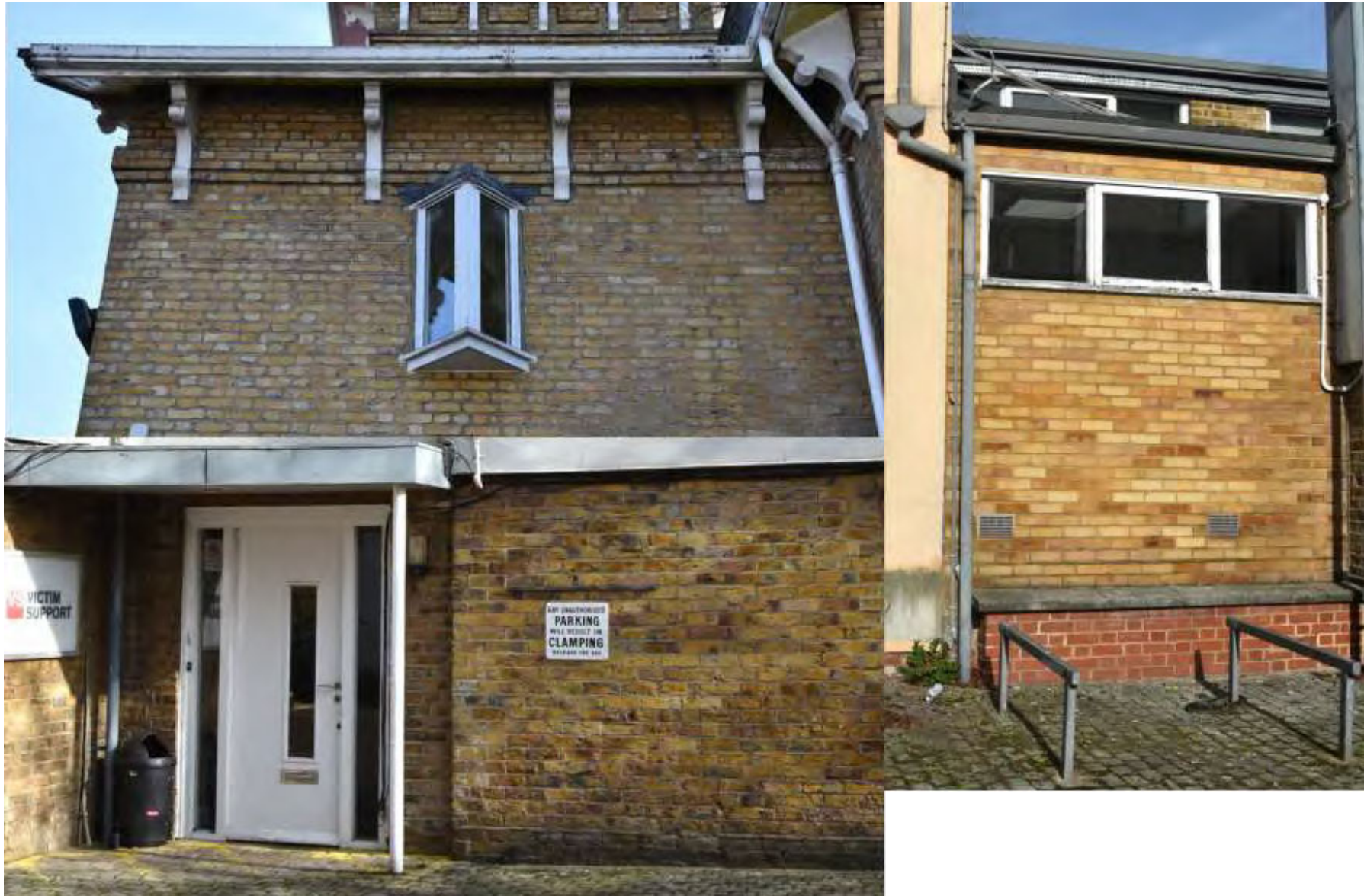
Figure 70: Examples of brickwork. Clockwise from top left: Victorian house with Flemish bond; 1960/70s corridor alongside hall with stretcher bond and Flemish bond; lower ground floor area occupied by Victim Support with stretcher bond.
