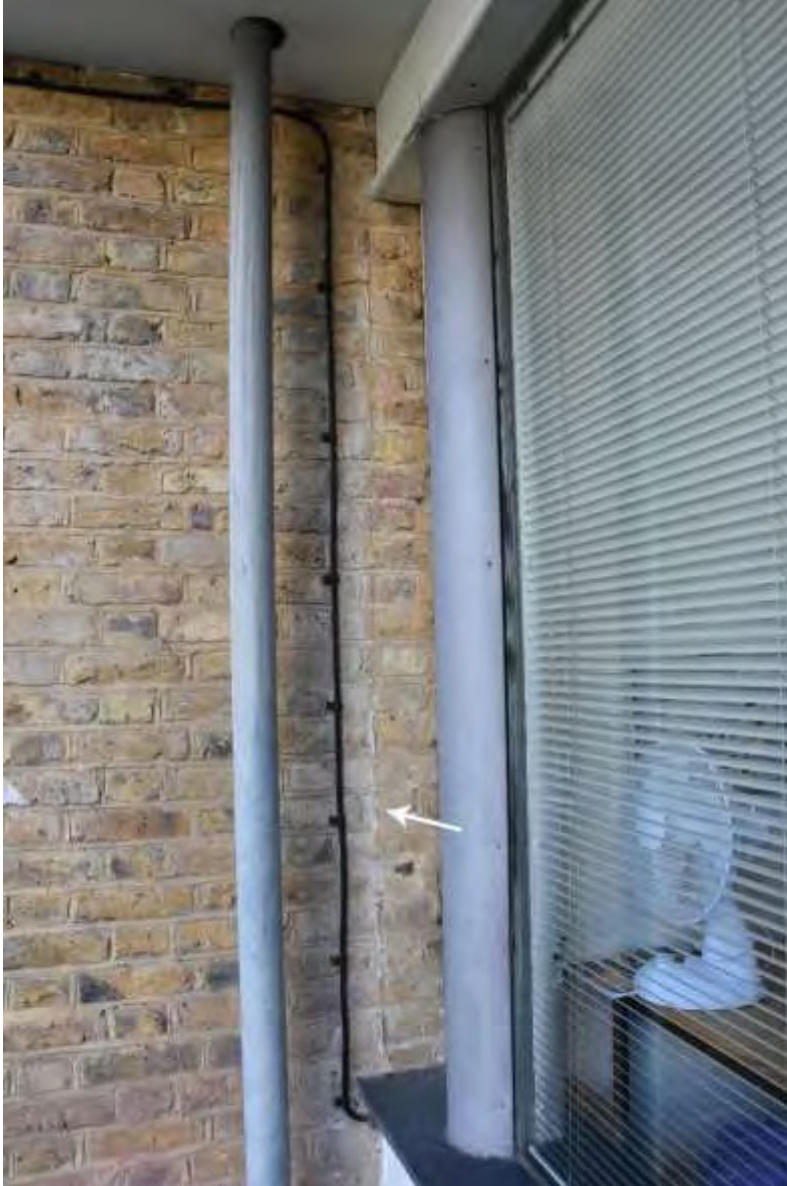
Figure 24: Detailed view of point 3 in Figure 23: scratches and remnants of white mortar on the exterior wall
