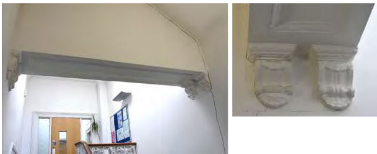
Figure 40: Original plaster corbels
