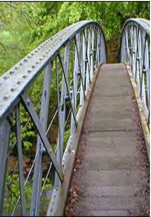
Open truss with rivet detail
