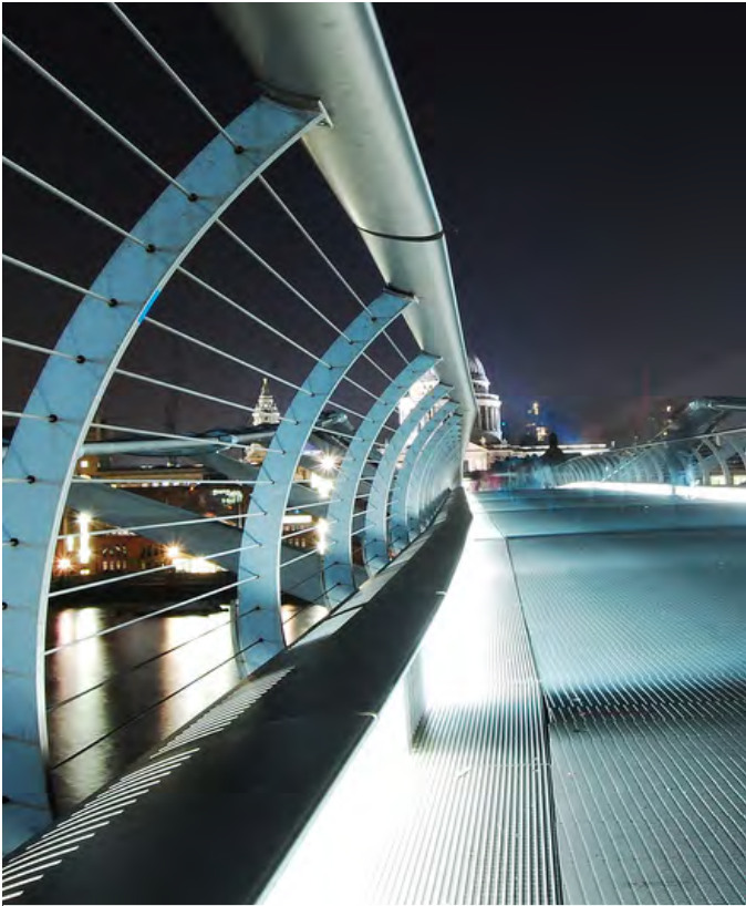
Lighting integrated into the bridge deck upstands washing the deck
