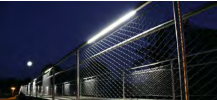
Lighting provided within the handrail
