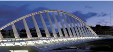
Lighting integrated into the bridge deck upstands
