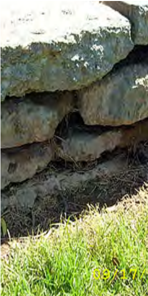
Reclaimed concrete retaining wall
