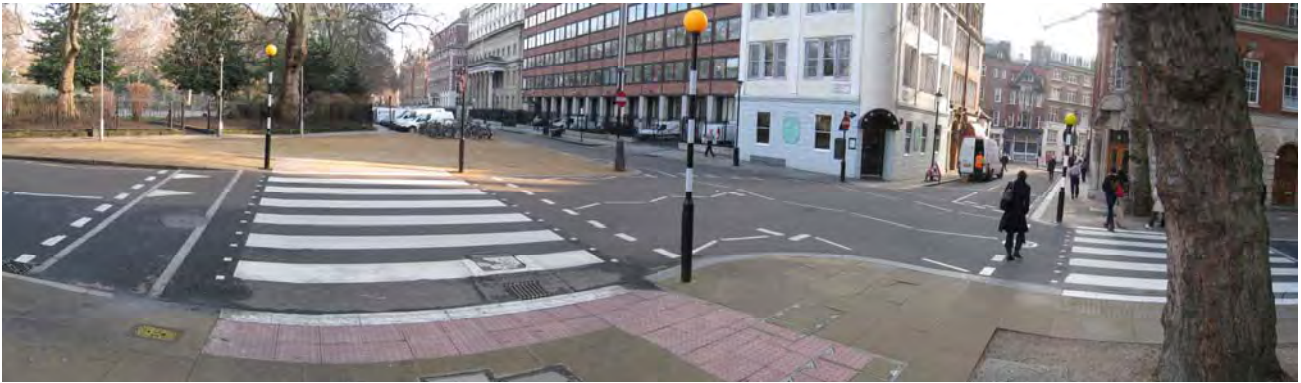
Figure 1: New pedestrian area on southwest corner of Lincoln's Inn Fields with a raised junction, two, new zebra crossings, and new park entrance.
