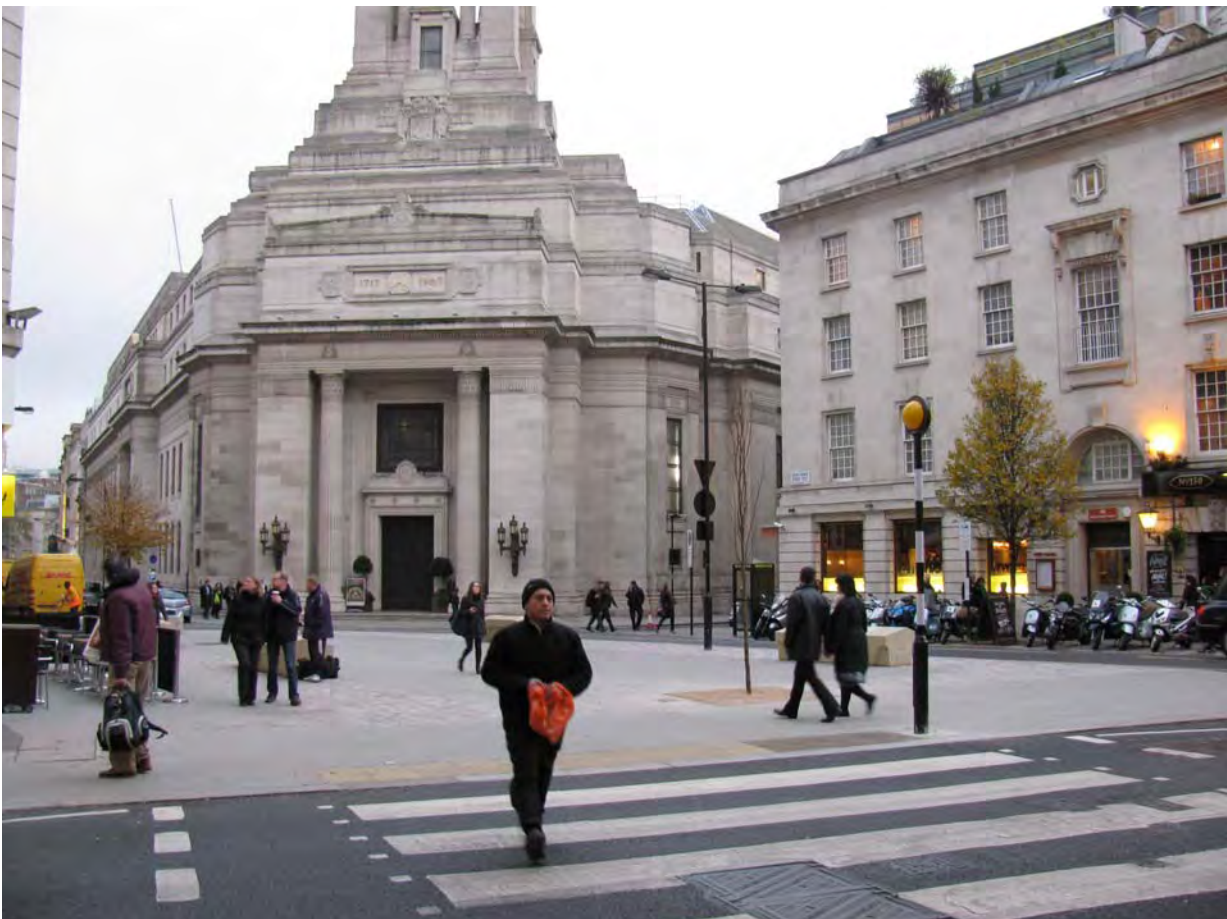
Figure 2: The new scheme created a shared space, a new public space, and wider footways to enable pedestrians to cross wherever is convenient.
