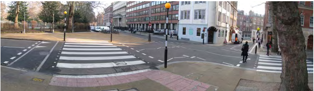
Figure 3: shows one of the new pedestrian areas with a raised junction, new zebra crossings, and new park entrance in to Lincoln's Inn Fields.
