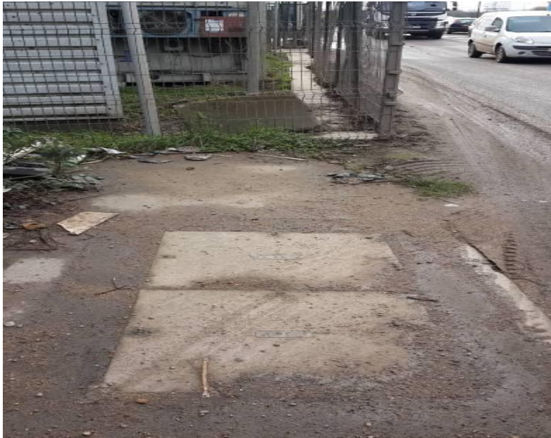
Pic 3.: BT chamber at end of the northern section of Hindmans Way. A road realignment (from this point) is required to ensure adequate space on both sides of the new highway for the footway / cycle path to avoid an existing building.
