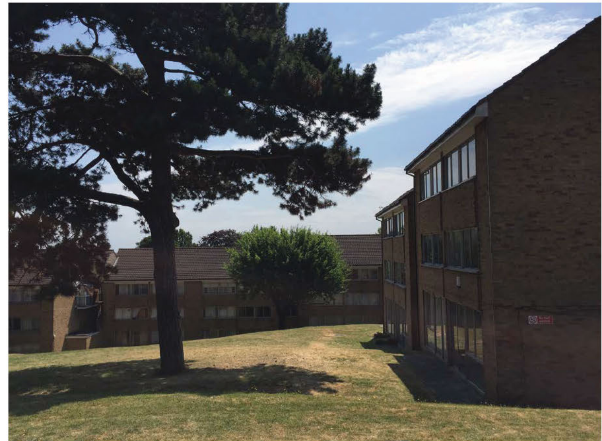
Middle terrace terrace
