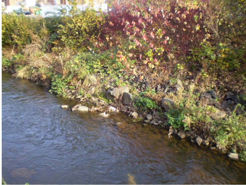
Photo 3 River Stour, Kidderminster Naturalised Rock Armour
