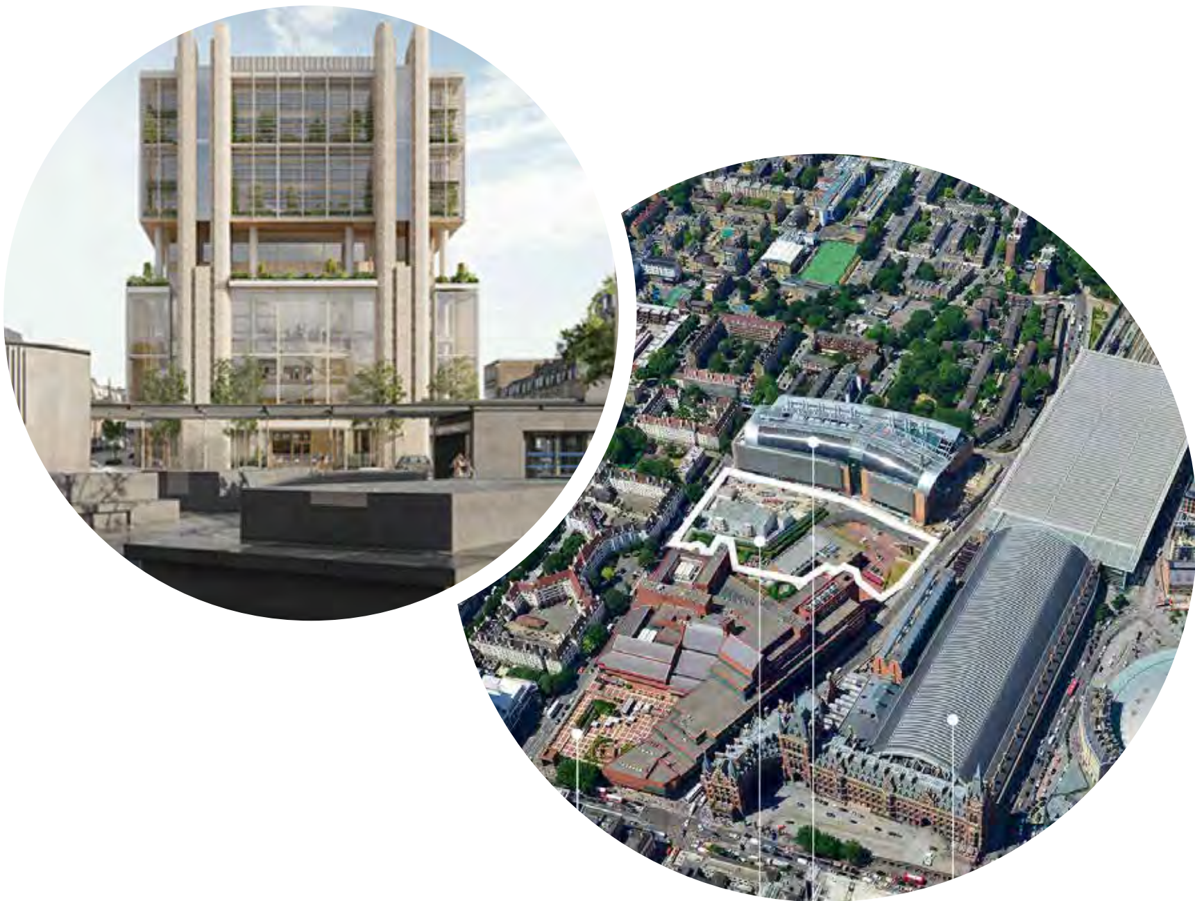
– MSD Discovery Centre – British Library Extension, St. Pancras
