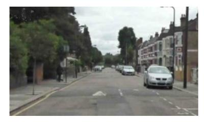
Above is a typical London road hump. The problem here is that it not only slows down motor vehicles but that it's abrupt changes in level are hazardous to cyclists. Ideally humps should be removed and the 20mph speed limit should be enforced. If not; this hazard should be reduced by making the hump a sinusoidal shape, the rise and fall are more gradual. Likewise the sinusoidal shape should be used at table, or raised, junctions.
