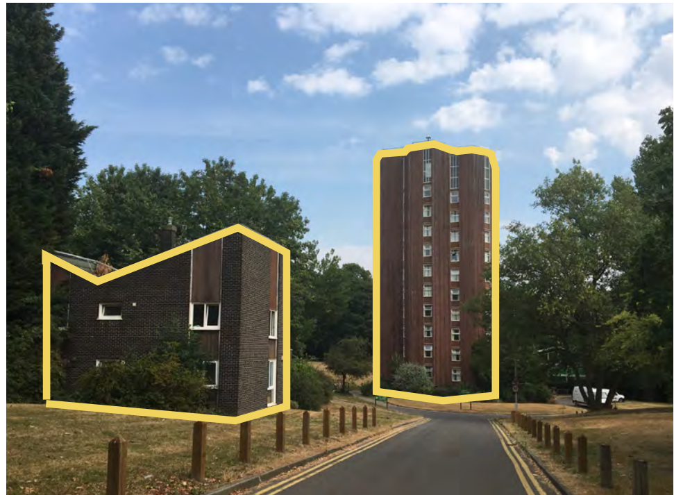
4. The Lodge and housing in poor condition and disrepair. Not appropriate infrastructure for park context.
