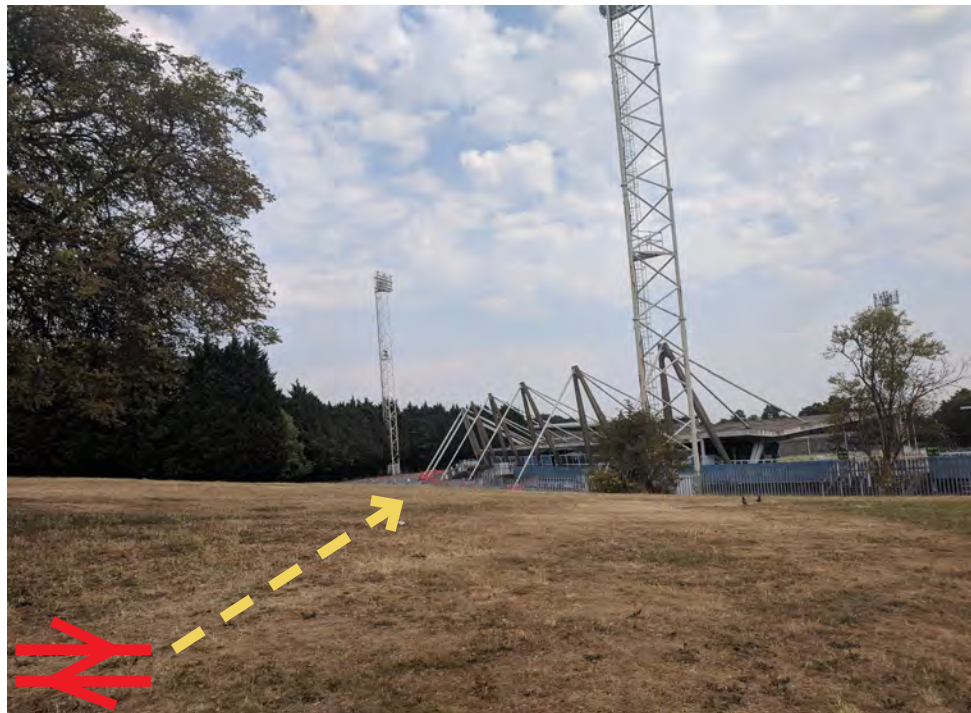
1. Lack of clear/ safe route to NSC site for pedestrians from Crystal Palace station.
