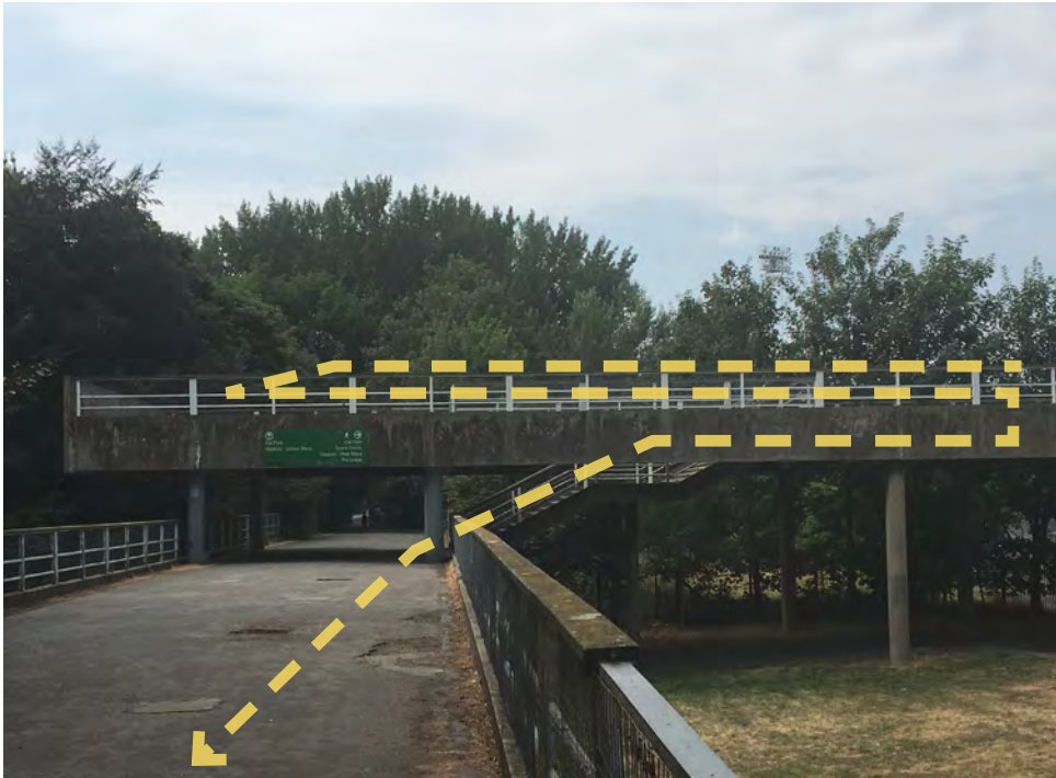
8. Unclear route/ connection of raised walkway to park.
