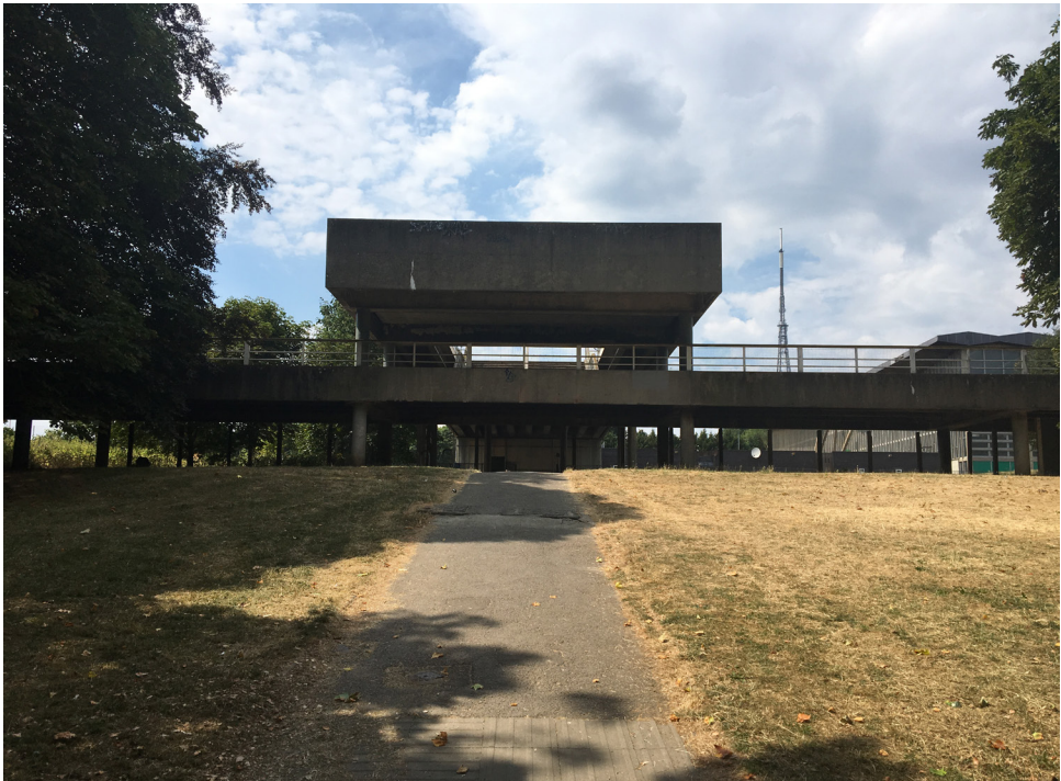
16. Raised walkway (Penge approach).
