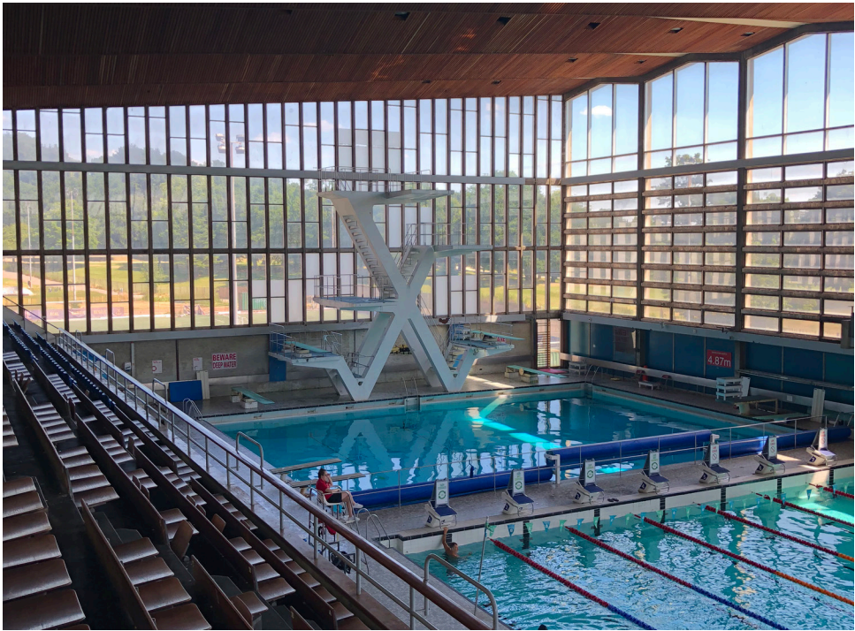
10. Pool and seating terraces.
