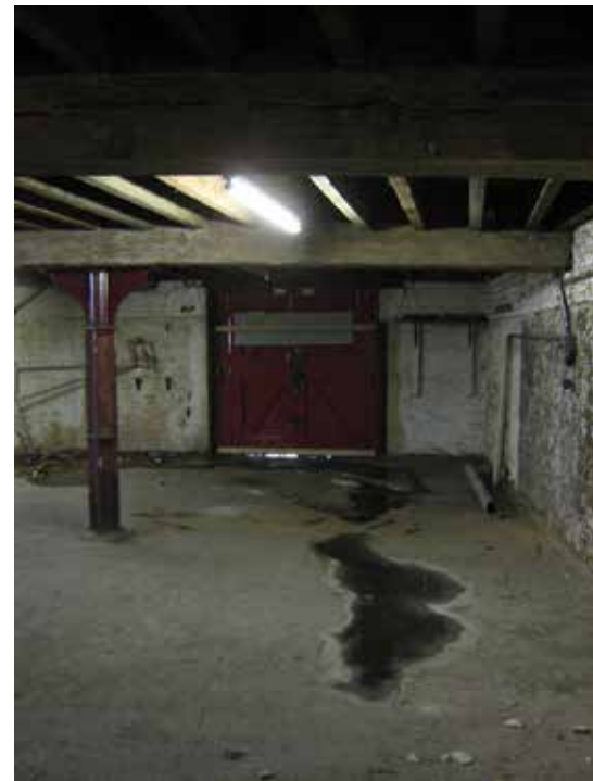
Figure 3. DOOR TYPE 1 - Typical original hatch rank timber boarded doors. DB1, DG3 & D2-2.
