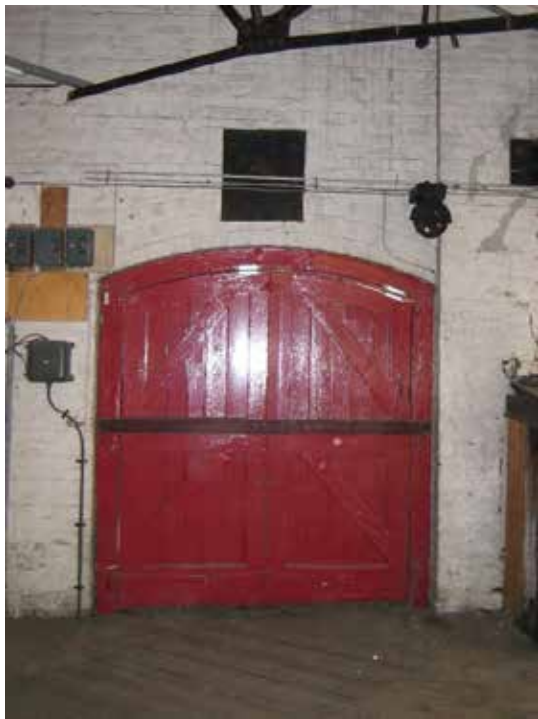
Figure 6. DOOR TYPE 4 - Typical original arched head hatched rank timber boarded concertina doors. D3-1 & D3-2.
