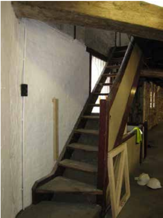
Figure 26. STAIR TYPE 1 – Original from ground floor to first floor. All enclosures modern.
