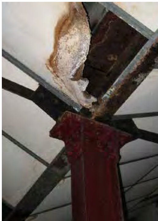
Figure 2 Figure 13. COLUMN TYPE 2 – 1940s rolled steel column to Third floor, supporting steel trussed.
