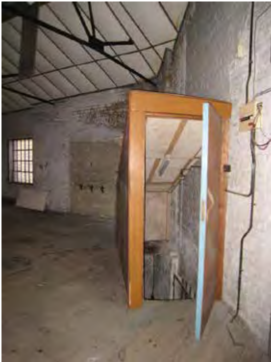
Figure 28. STAIR TYPE 1 – Original from second floor to third floor. All enclosures modern. Stair type the same – condition varies floor to floor.
