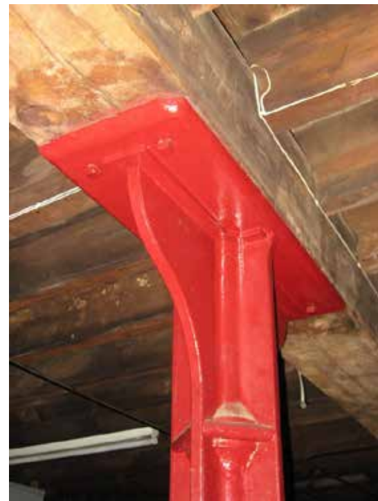
Figure 1. COLUMN TYPE 1 - Typical original cast iron column to basement, ground, first and second floors.
