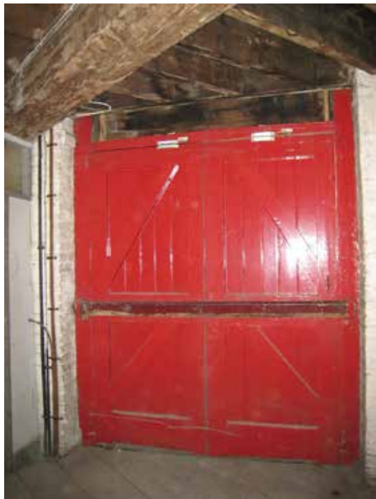
Figure 5. DOOR TYPE 3 - Typical original hatch rank timber boarded concertina doors. D1-1, D1-2, D2-2, D3-2 & D3-1.
